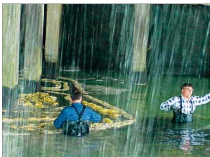
Compound fibers REO Fb have been used for the removal of hydraulic oil from the cooling stack pool of electric plant
