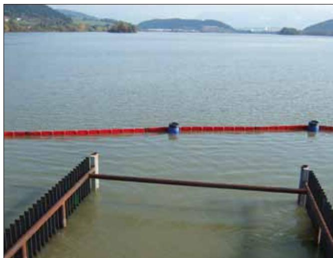
Whole year long protection of small water power plant gating. Containment boom REO758 avoids settlement of floating pollutions.
