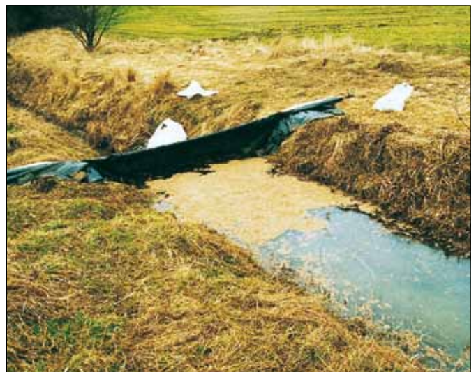
During the construction works on the water stream, it is possible to use the dam barrier for the water transfer over the building site. It can also be used during the building and rebuilding of the bridges, canal locks, pillars, crossings of other line constructions across the water (gas pipeline, water pipe, canalization, oil pipeline or product pipeline). Metal sleeve ring is easily removable.
