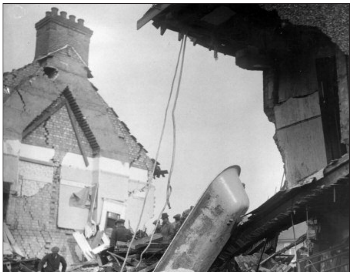
Damage in De Bohun Road, Southgate, February 1941. Picture courtesy of Local History Unit.
