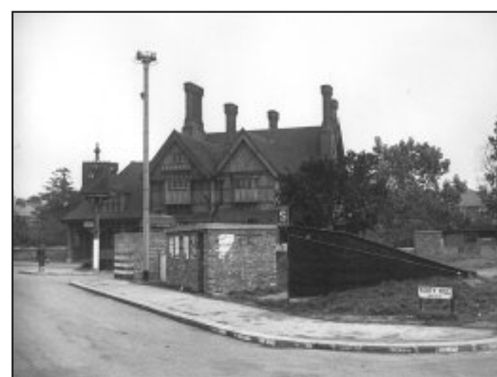
Surface shelter and air-raid siren outside The Goat public house, Forty Hill. Picture courtesy of Local History Unit.
