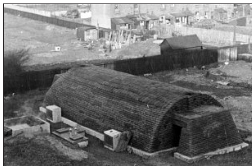
Tottenham and District Gas Company Gas, Emergency booster plant at Ponders End. The building is covered in sand bags for protection. The Enfield Gas company had been taken over by the Tottenham and District gas company (based on the Tottenham / Edmonton border in Willoughby Lane) in 1914. An unusual use of their town Gas was a co-operation between RAF balloon command laying pipes to top up barrage balloons. Tottenham and District Gas Company. Experiences during War Period. Photograph courtesy of Local History Unit.
