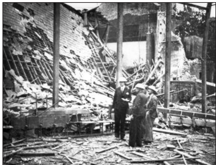
Inspecting the damage at the Alcazar cinema and dance hall, Fore Street, Edmonton the morning after the raid on 23 August 1940. Picture courtesy of Local History Unit.
