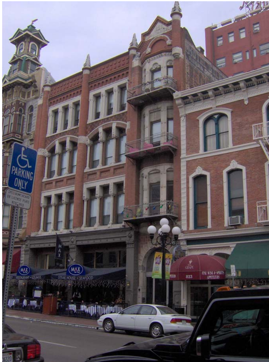
Figure 15. Greely-Nesmith Building, 2006 Source: Author
