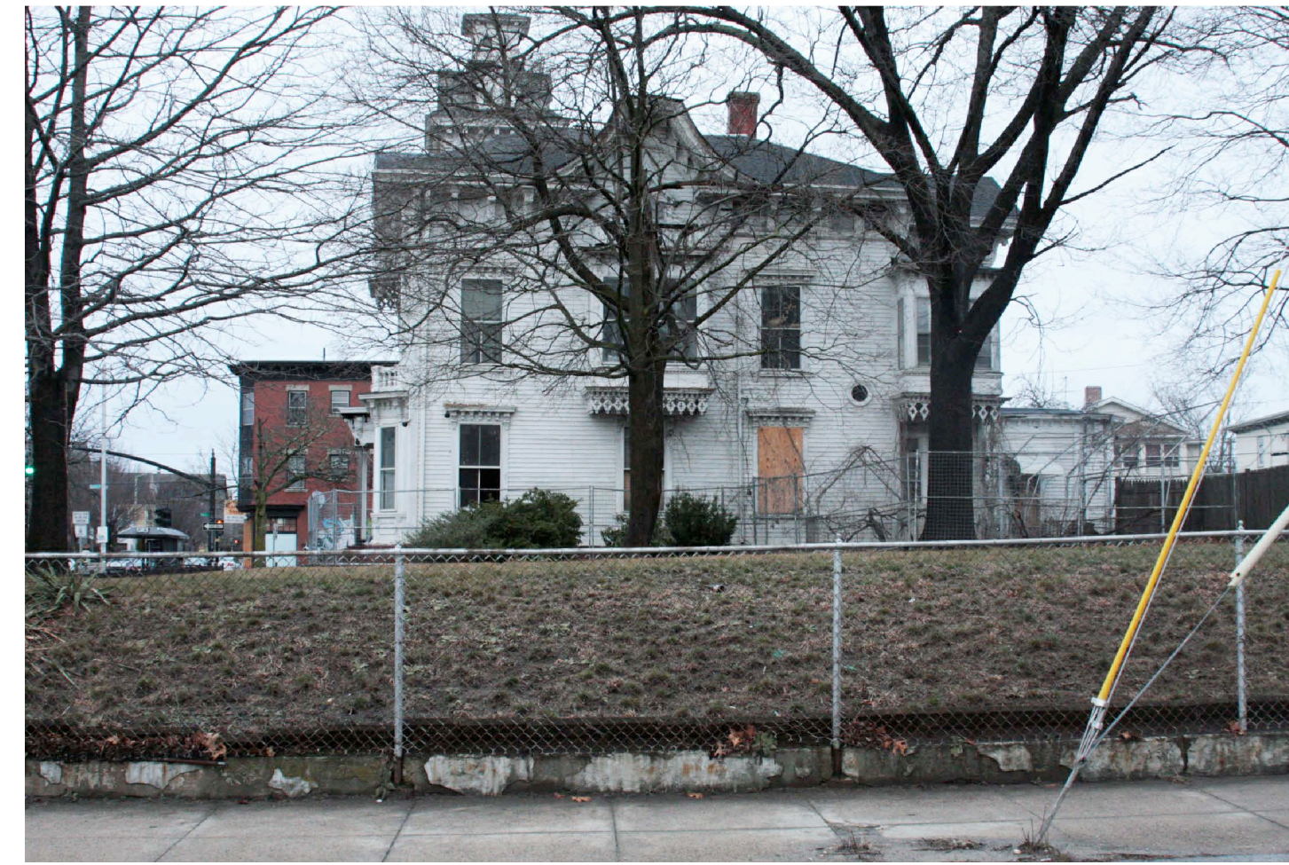
EAST ELEVATION (FACING BAINBRIDGE AVENUE)
