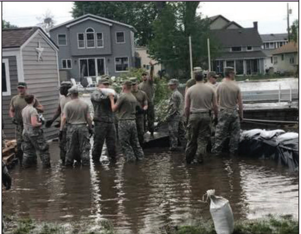
New York Army National Guard 105th Military Police Company Soldiers construct a sandbag barrier to protect property at Sodus Point, N.Y. from flooding due to rising waters on Lake Ontario on May 22. Photo by Sgt. 1st Class Patrick Belmont, 105th Military Police Company.
