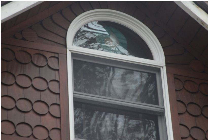
Gable detail, north facade Sarah Moses (LPC), 2017
