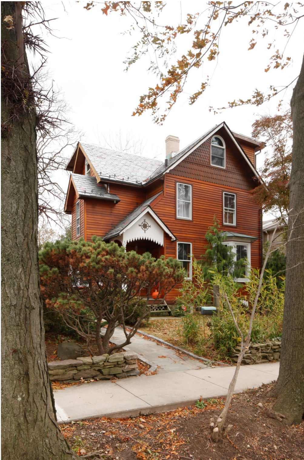
Samuel H. and Mary T. Booth House 30 Centre Street Sarah Moses (LPC), 2017
