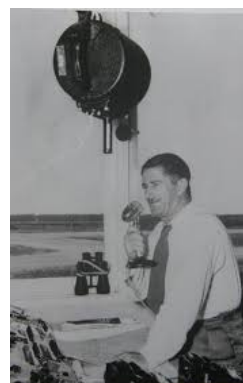
'Jack' Buckham Adelaide Control Tower 1955 Photo courtesy website '5DME' accessed 3 rd Aug 2016
