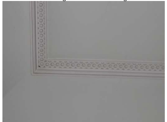
Img. 16 detail of ceiling cornice in main hall
