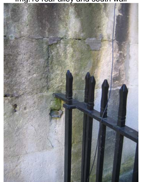
Img.12 remains of original railing
