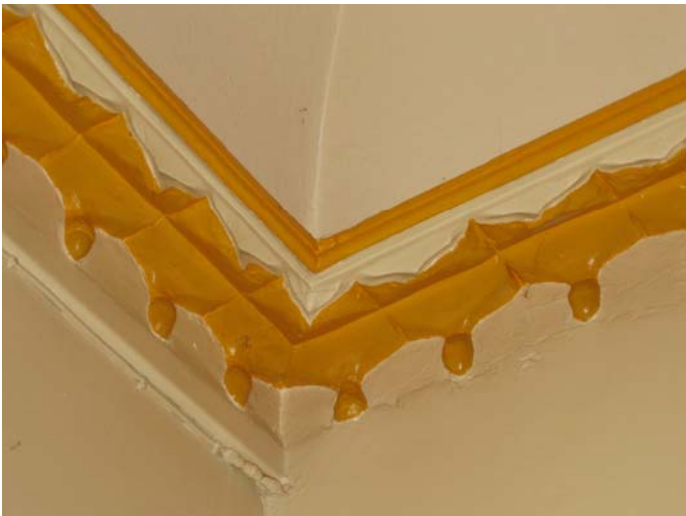
Img. 36 detail of basement cornice
