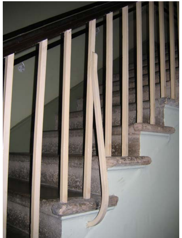
Img. 28 detail of staircase fixing rods
