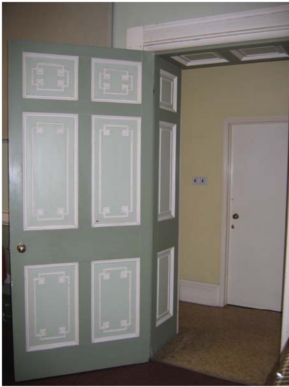
Img. 19 doorway in south-east corner of main hall
