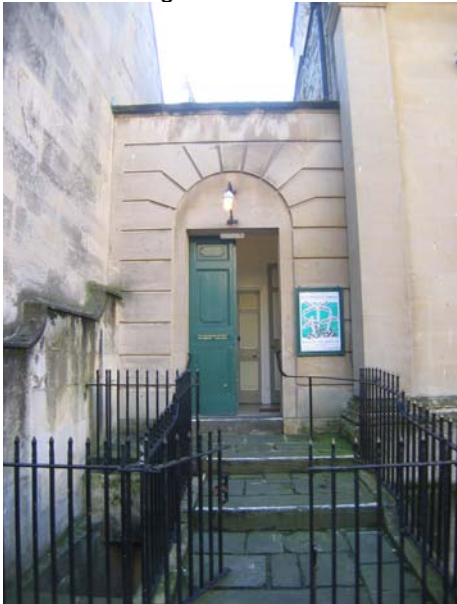
Img. 3 east entrance
