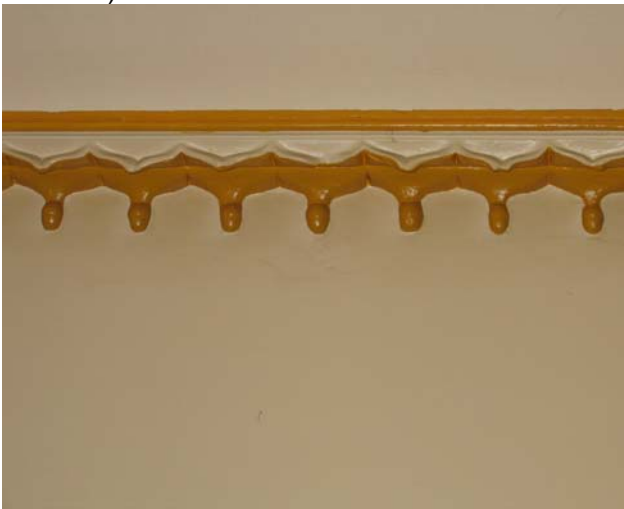
Img. 35 detail of basement cornice
