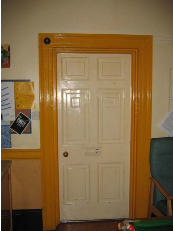
Img. 33 Door into 'Tylers Room' (Ante-Room 2) north-west corner of basement
