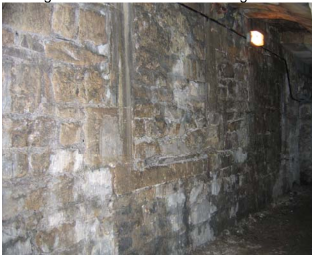
Img. 47 north wall with blocked window
