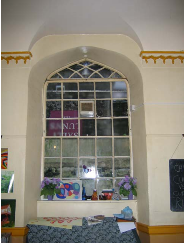
Img. 34 Central Gothic window in south wall of basement
