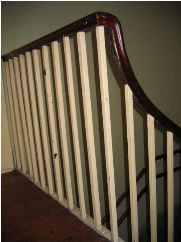
Img. 27 Top of staircase
