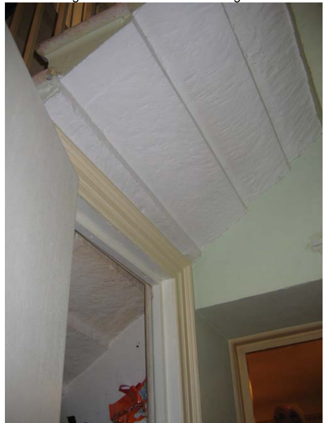
Img. 30 area beneath the staircase
