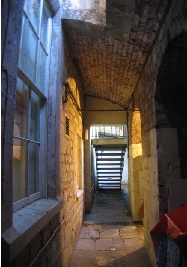
Img. 45 area at north front looking west
