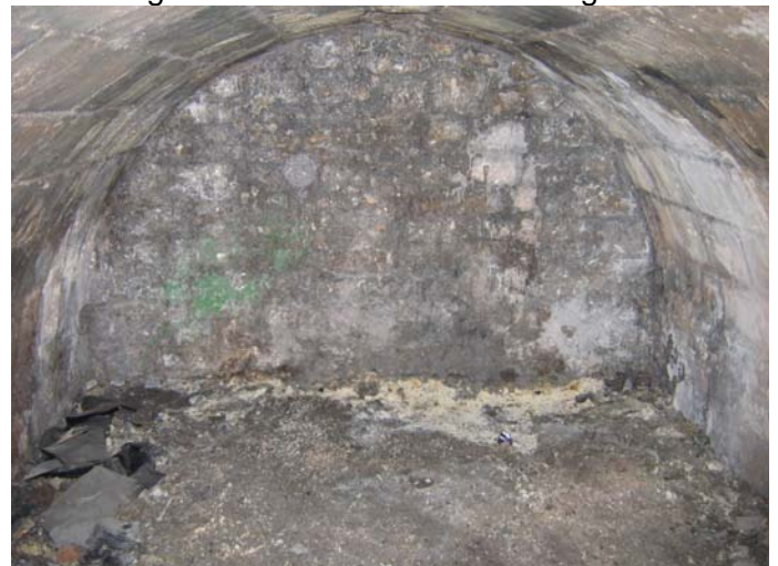
Img. 48 one of the vaults
