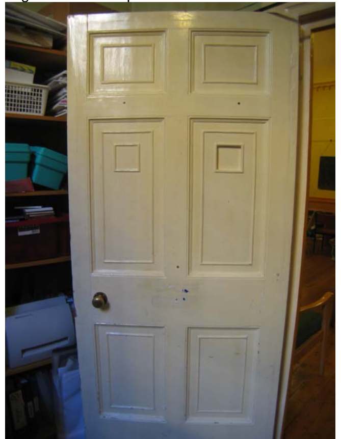
Img. 40 detail of Ante-Room 2 door with peephole
