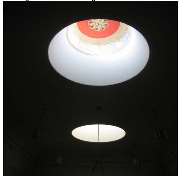
Img. 18 the two roof lanterns
