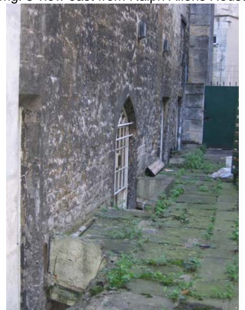
Img.10 rear alley and south wall
