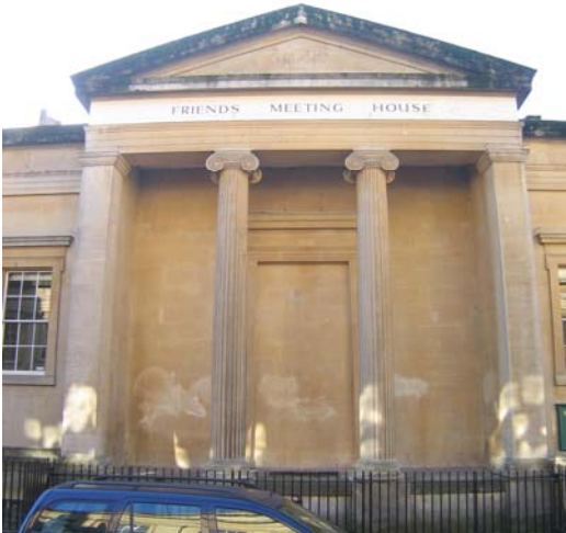
Img.1 North front
