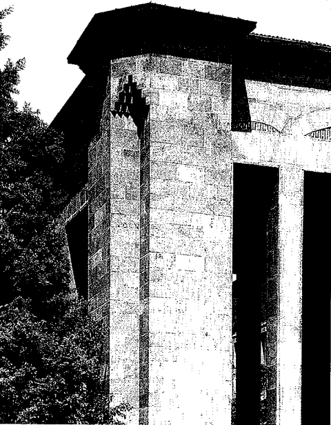
Corner detail of the entrance portico with the muqarnas motif Photographs: Atelye Mat
