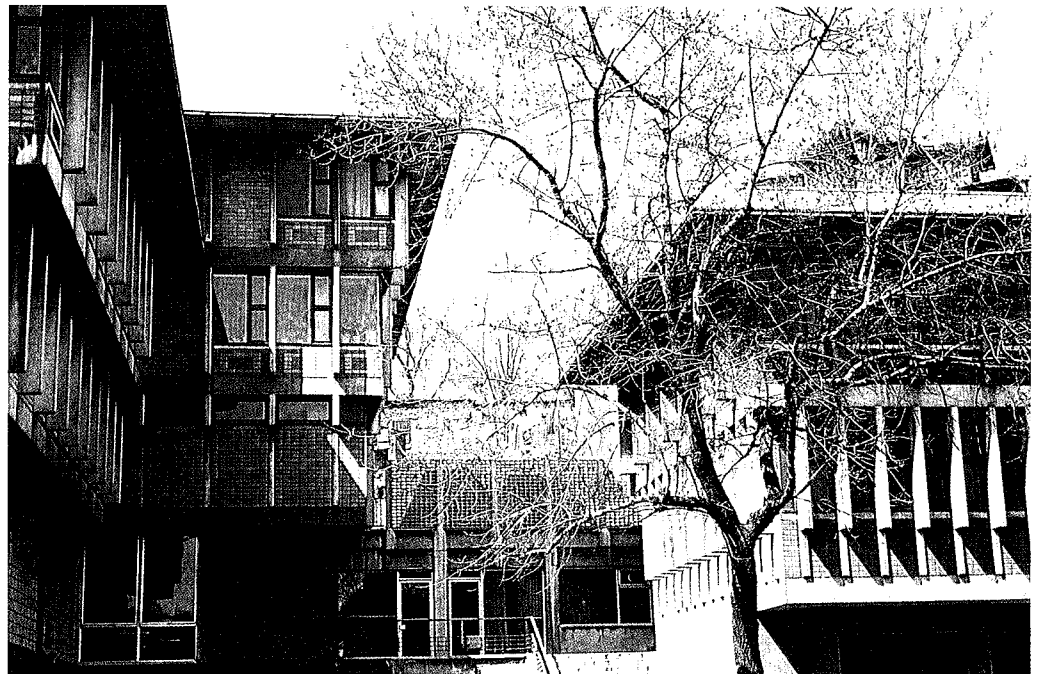
Each floor is cantilevered out slightly above the lower floor Photographs: A Dündar/AKAA
