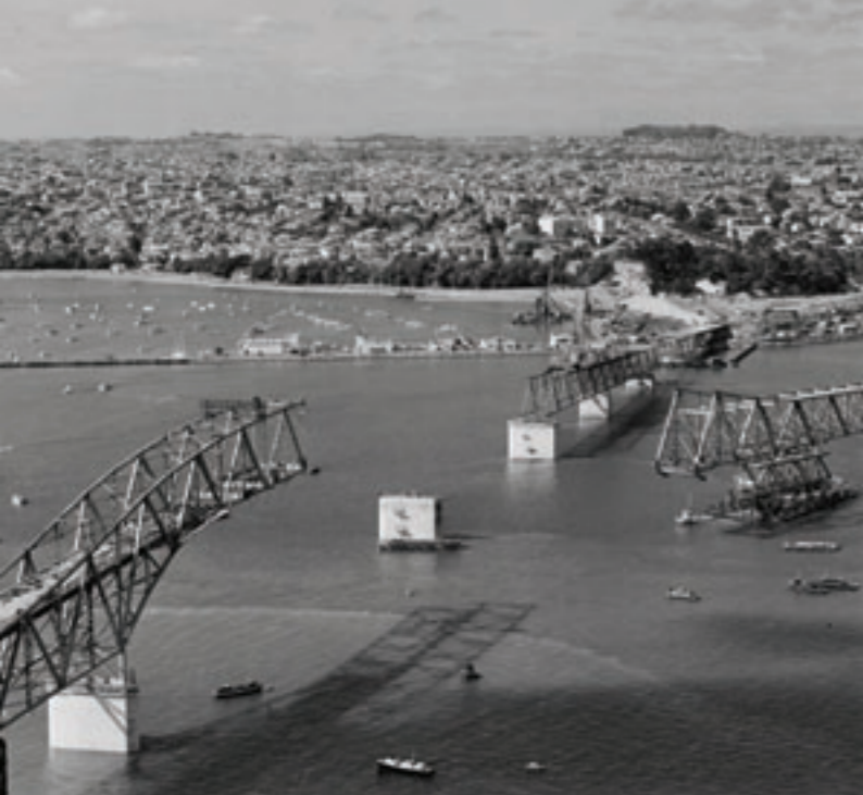
12 Auckland Harbour Bridge construction
