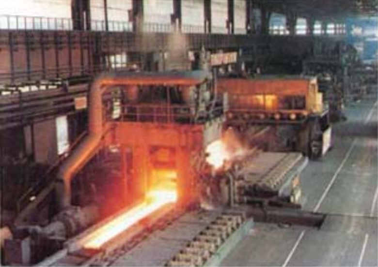
The hot rolling shop of the Kim Chuck Iron and Steel Complex
