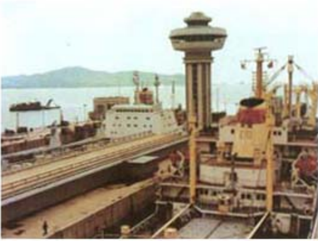
A ship passing through a lock of the West Sea Barrage
