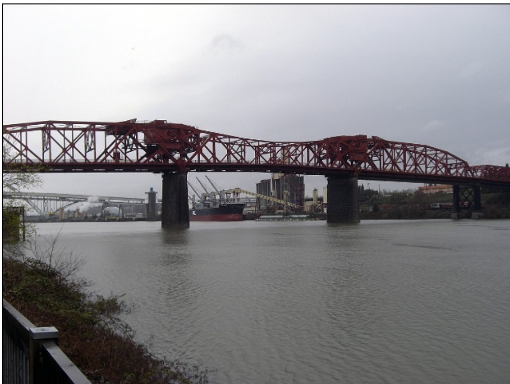
Photo 4 of 4: (OR_MultnomahCounty_WillametteHwyBridgesMPD_BroadwayBridge_0004) Downstream view, Operator's tower
