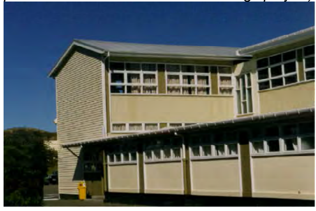
Overview rear oblique (Tawa College Block C photo from Aurecon standard buildings project)
