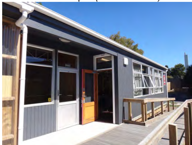
Overview rear oblique (AGHS E Block)
