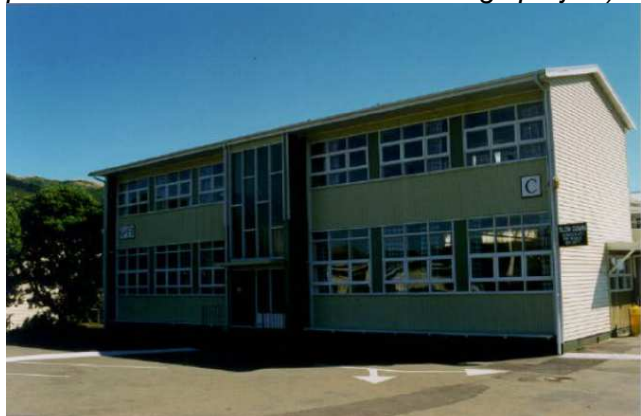
Overview front oblique (Tawa College Block C photo from Aurecon standard buildings project)
