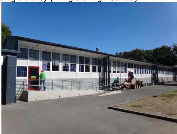
Similar appearance but based on 1950's block single storey ( Rangiora High School )
