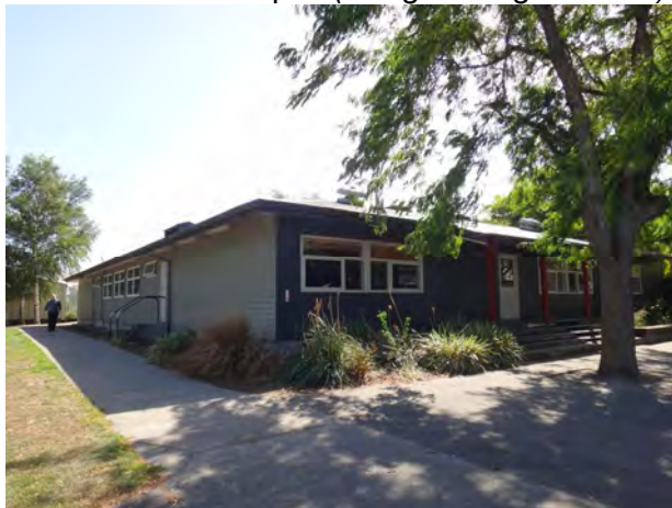
Overview rear oblique (Rangiora High School)
