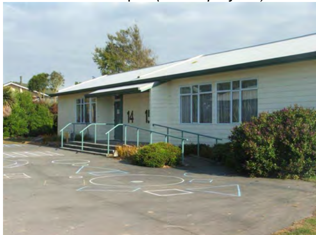
Overview front oblique (West Spreydon)
