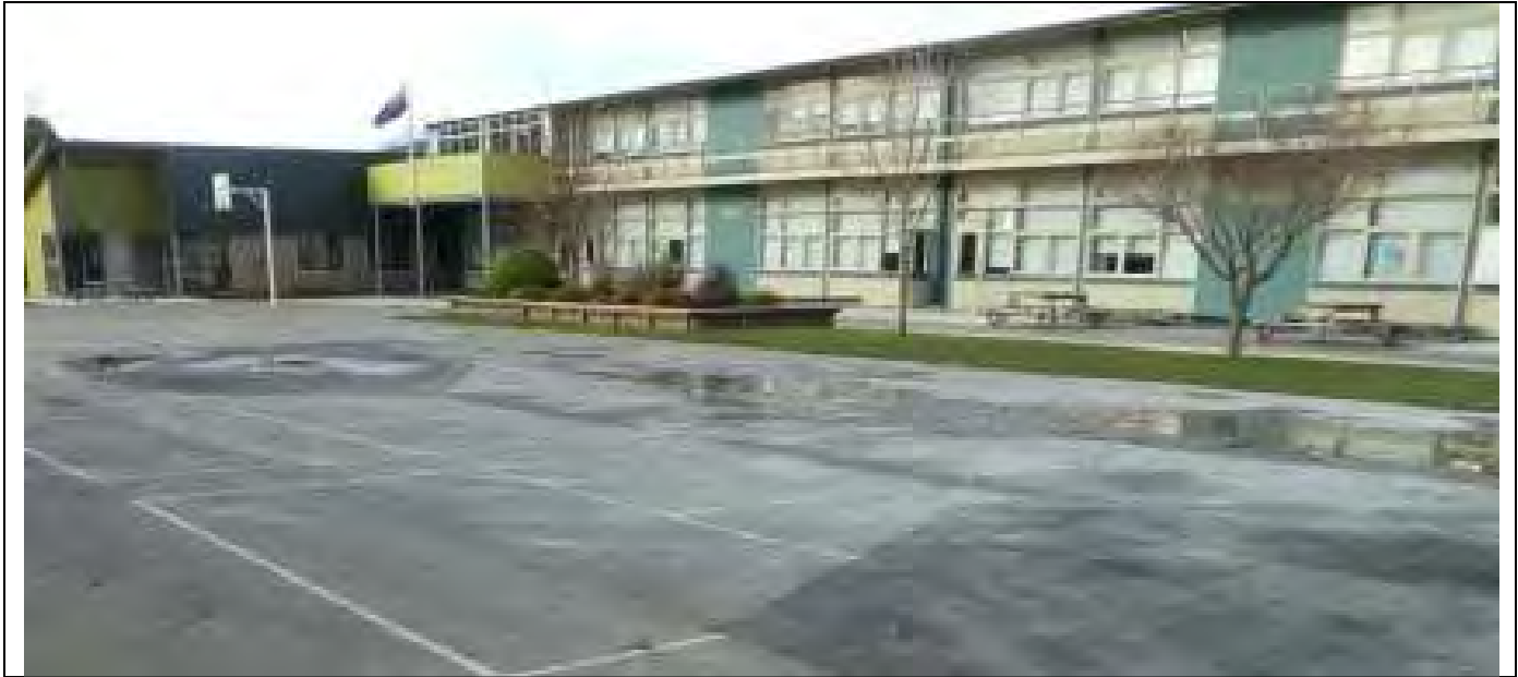
12 Classroom Two Storey Block
