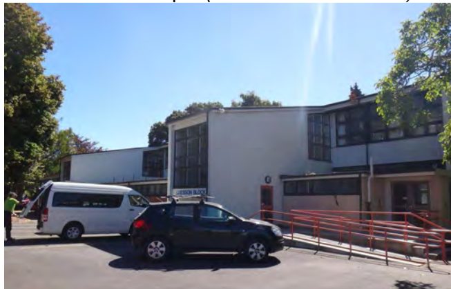
Overview rear oblique ( Gresson Block AGHS )
