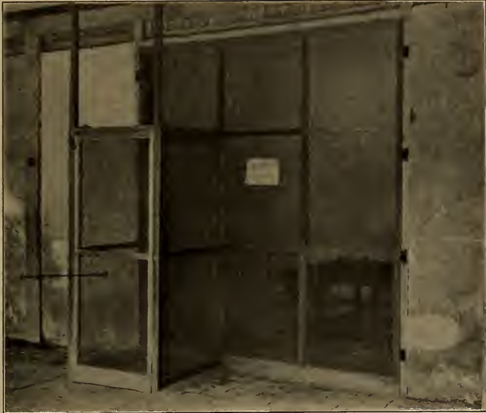
Fig 1. Screened compartment at factory; a, one of the two screened doors with screened vestibule.
