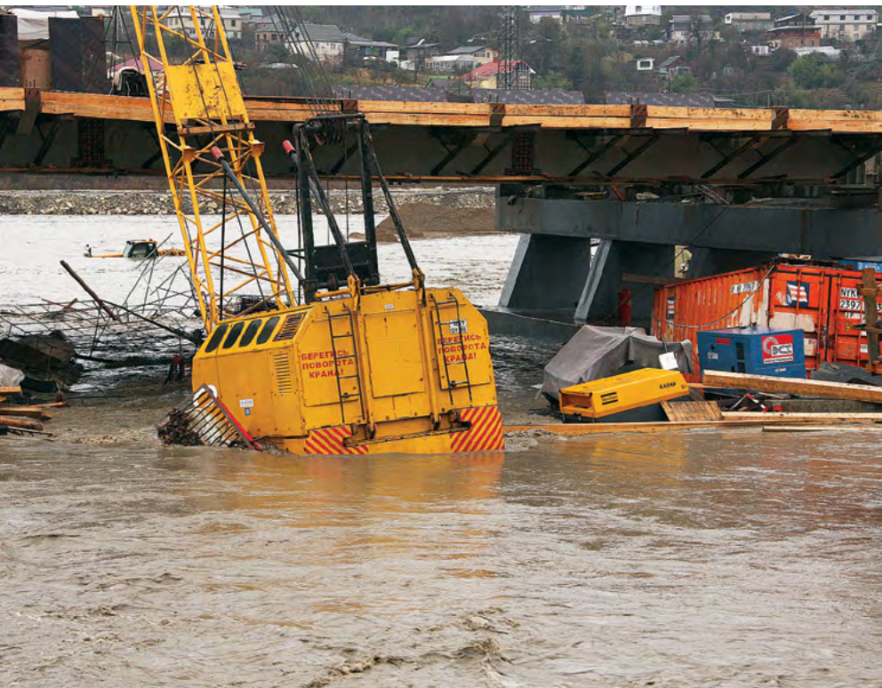
Equipment inundated in the floodplain of the Mzymta River on 29 December 2009
