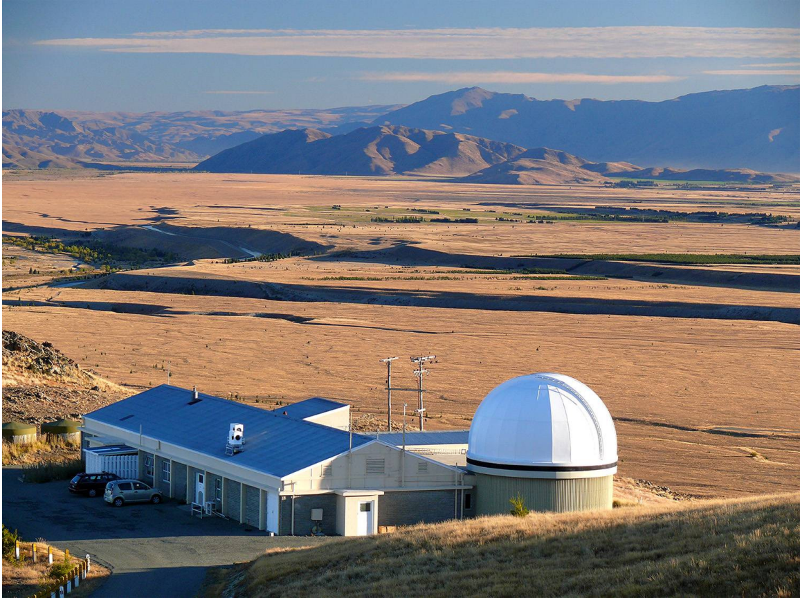
1.0-m McLellan telescope dome and accommodation building at Mt John
