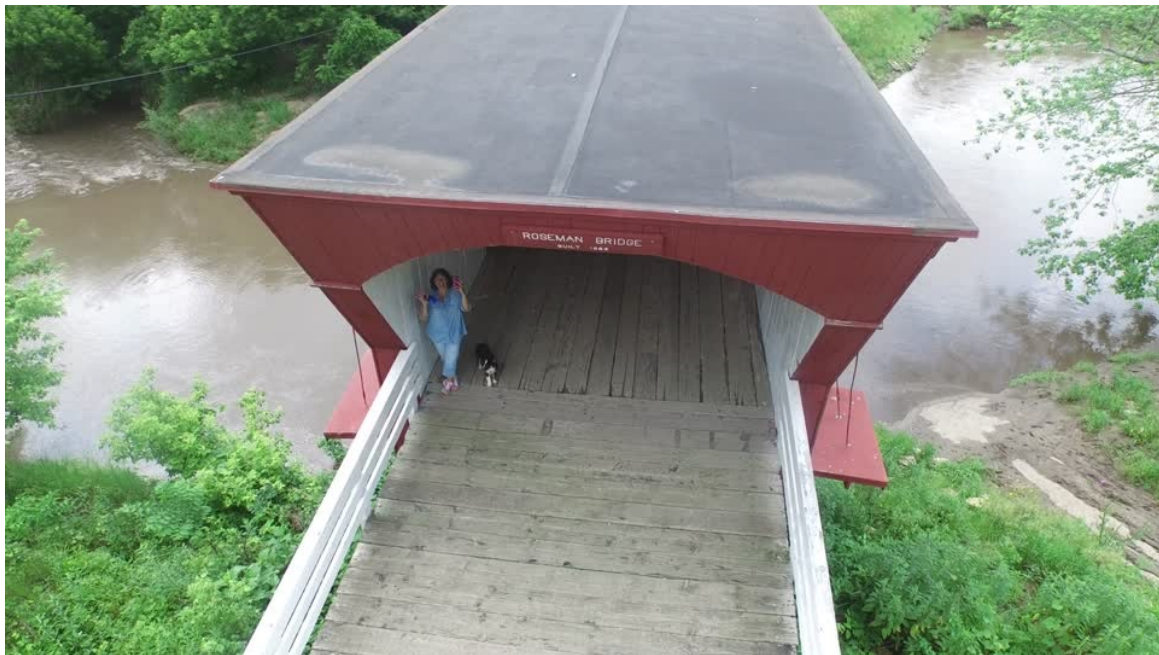
Figure 36: Roseman Bridge sequence, frame 25
