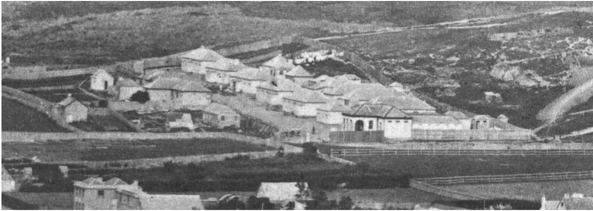
Figure 10: Detail of Stock's photo, showing the Lower Barrack sin the area of what is now Buckle St
