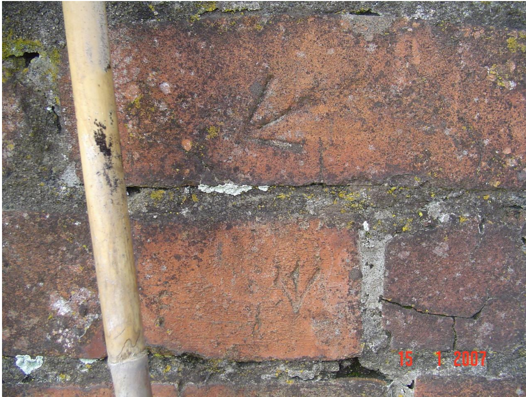
Figure 22: Prison brick, wall at Government House, Wellington
