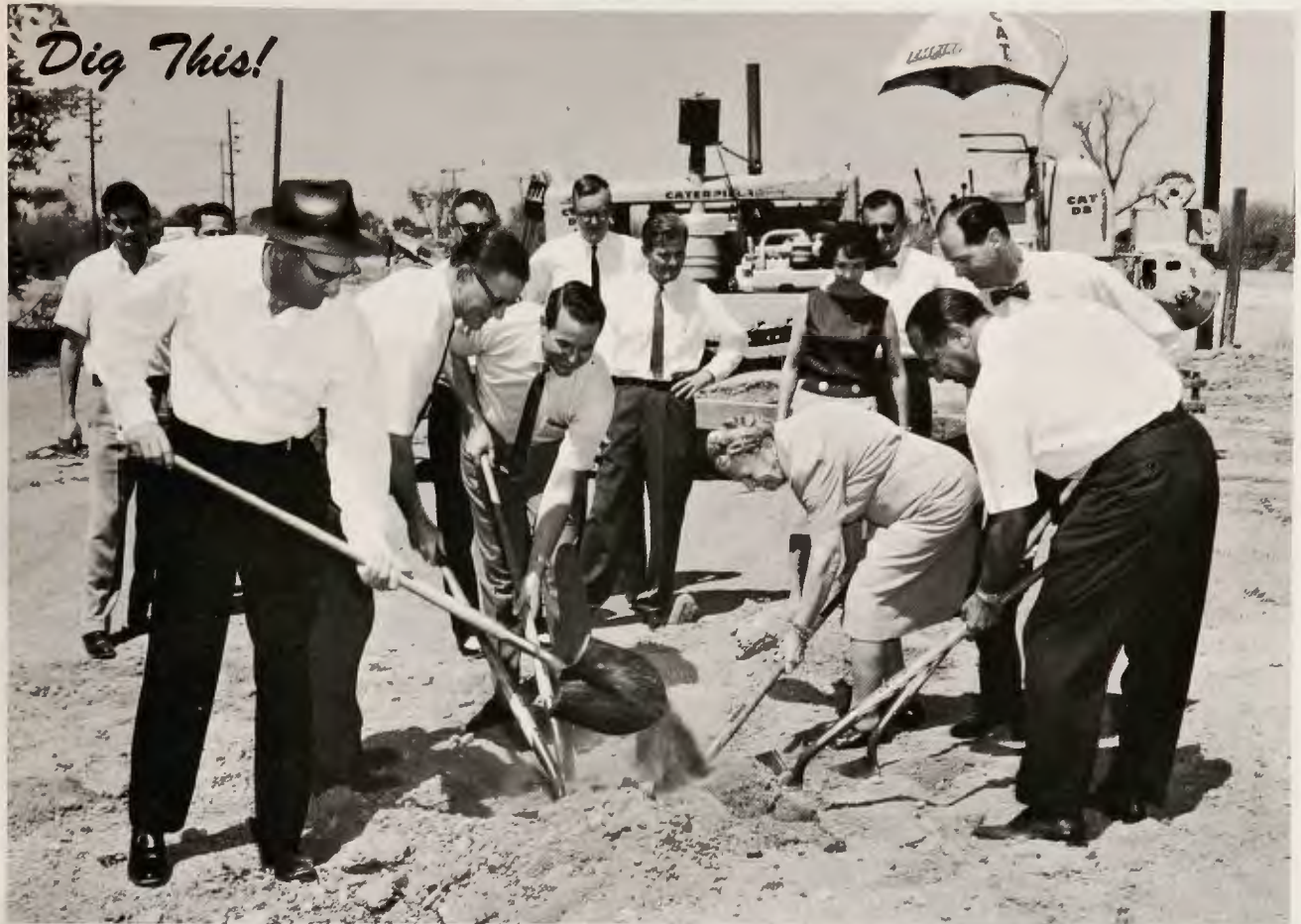
'A LOT OF HIGH-PRICED TALENT' , opined Project Supt. Fred McDowell as this group took over the ground-breaking project which formally launched construction of Webb headquarters at the multi-million dollar Rosenzweig Center in Phoenix. From left: Pres. Del E. Webb, Executive Vice-Pres. L. C. Jacobson, Richard Wartes of Webb Corporation, Mrs. I. Rosenzweig, 81, "queen" of the ceremonies, and her two sons, Newt and Harry Rosenzweig, brother jewelers and owners of the valuable 12½-acre North Central Avenue site of Rosenzweig Center.
