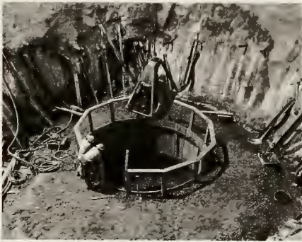
Clamshell excavates dirt and rock loosened by powder charges.
