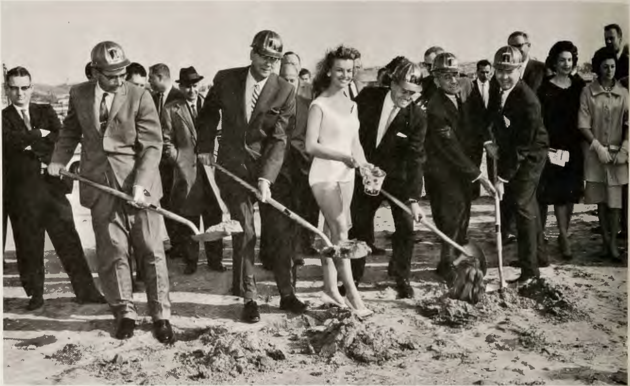
SANDY SOIL on which new Del Webb's OceanHouse hotel will rise beside San Diego's Mission Bay provided comparatively easy digging for groundbreaking principals who got construction officially under way last month. In action with shovels, above, from left, are: Douglas Giddings, chairman, Mission Bay Park Commission; Builder Del Webb; Charles Dail, San Diego mayor; Archie Loveland, OceanHouse general manager, and Richard M. Wartes, Webb vice-president and manager of the commercial and industrial division. Turning a sandbucket spadeful is Sharon Wetzel, Miss Pacific Beach, representing the year-around appeal of San Diego County and the Mission Bay area.
