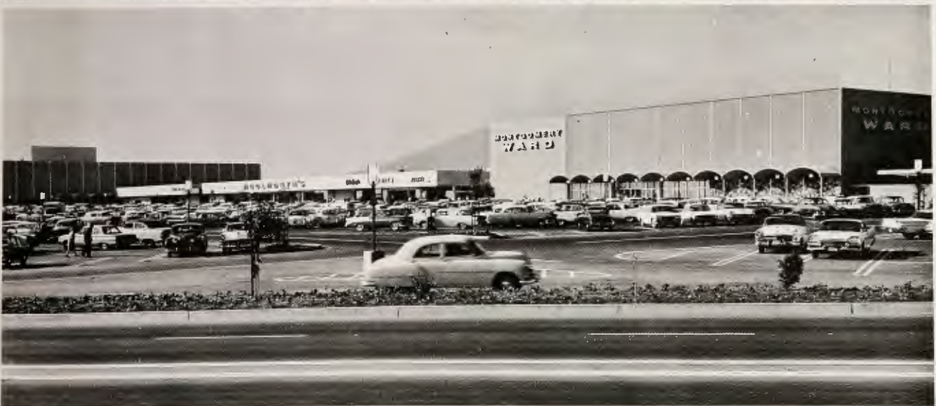
MONTGOMERY WARD store shown in photos above, is similar to Ward's store in Chris-Town Center in Phoenix. Ward's in Grossmont, as one of two key center tenants, occupies 122,000 square feet of retail space. Showcase windows provide spectacular lighting display after dark.
