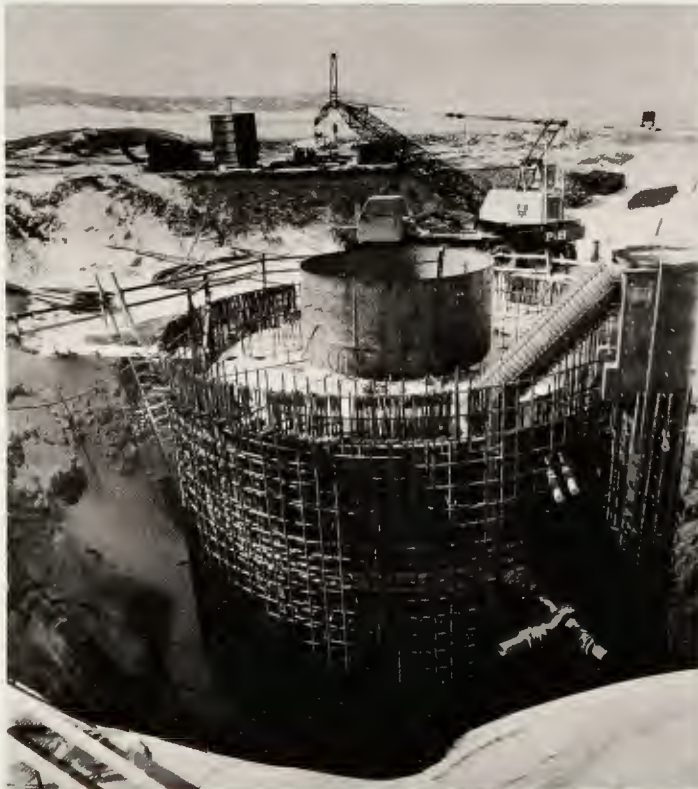
ALL THAT REACHES ground level of the missile silo is large round opening through which Minuteman is fired, and the smaller round opening which is access shaft for technicians.
