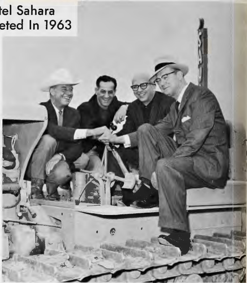
PLENTY OF TALENT was at the controls for the official ground-breaking to launch construction of the 24-story skyscraper addition to Hotel Sahara at Las Vegas, Nevada. Pictured above, from left: Rex Bell, Nevada's lieutenant governor; Alex J. Shoofey, Sahara-Nevada Corporation executive vice-president; Milton Prell, Sahara-Nevada president, and Dell E. Webb, Webb Corporation president.
