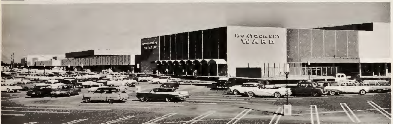
SOUTHWEST'S LARGEST and one of the nation's most modern shopping facilities, this huge Chris-Town Center at Phoenix is being pushed to completion by Del E. Webb Corporation workmen for an August 24 opening. It will have 55 stores and shops, parking for 5,000 automobiles, and will be owned and operated by the Webb Corporation.
