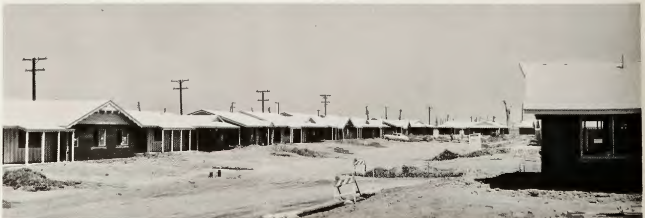
BIRTH OF A COMMUNITY — Houses now, but homes in a few short weeks when residents move in, this street in Del Webb's new Sun City, Calif. retirement community will soon take on a "lived in" look. New homes and apartments are being started at the rate of 12 per day. Webb builders install streets and sidewalks, and landscape homes before delivering them to buyers.
