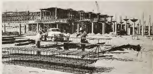
STEEL SUPERSTRUCTURE for 48 shops centered between Ward's and Marston's stores at either end of Grossmont structure is shown at left. Above, steel workers prepare reinforcing rods for columnar supports. Project calls for 1,200 tons of steel and 25,000 yards of concrete.
