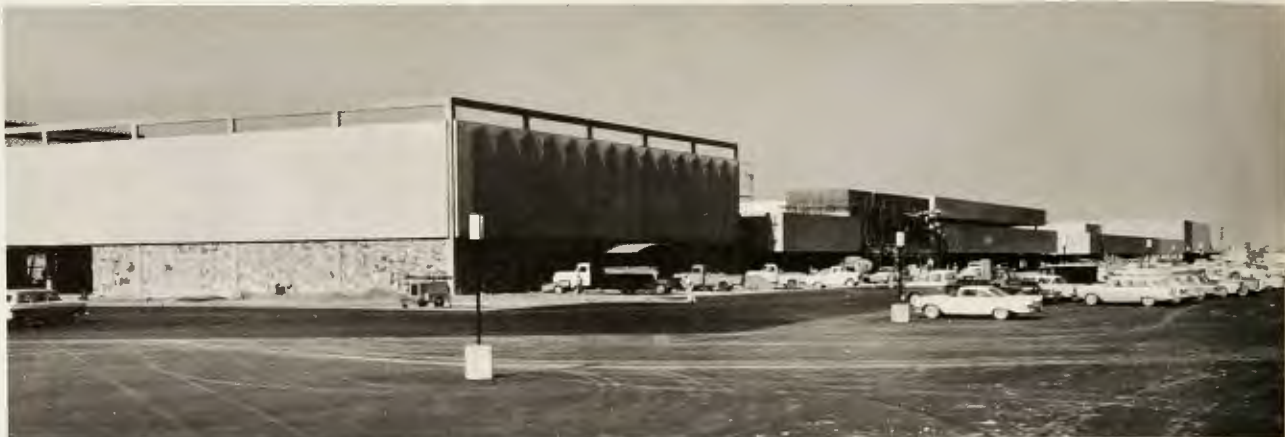
SOUTHWEST'S LARGEST shopping facility, Chris-Town Center at 19th Avenue and Bethany Home Road in Phoenix, pictured above, is heading for an official opening of its 50-plus stores and shops during the last week in August as Webb crews push interior construction. View above looks west, from Korrick's department store in foreground, along the Bethany Home frontage, several blocks in length. Inside, running the length of the center, will be a spacious air-conditioned shopper's mall, cooled in summer and heated in winter.
