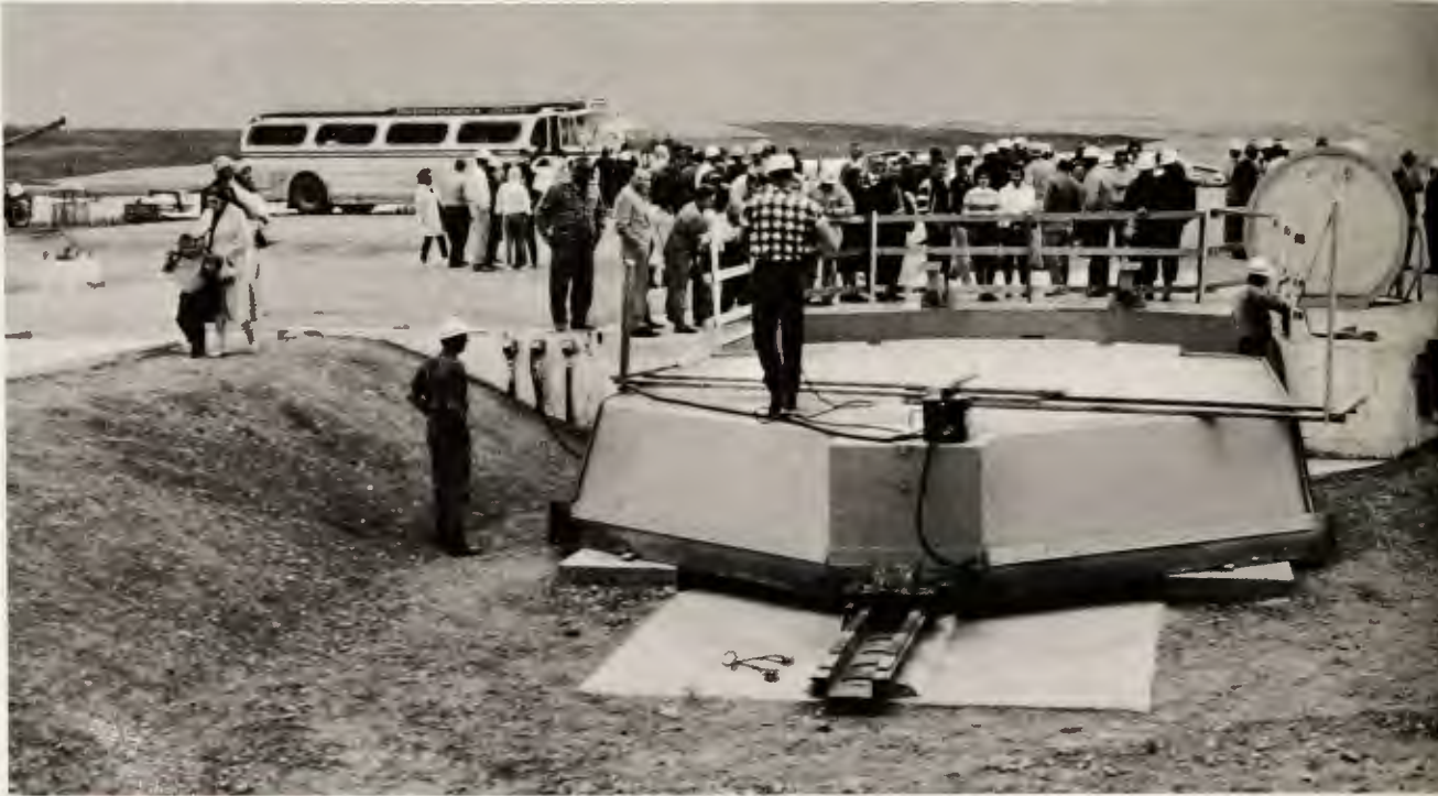
AT GROUND LEVEL of a Minuteman missile-launching site, there isn't a lot for visitors to see — simply the concrete silo cover in foreground, and the access shaft and escape hatch (with round steel lid) for missile technicians.
