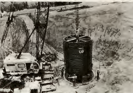
Weighing 25 tons, more than 13 feet in diameter, "barrel" is eased to silo bottom 82 feet below ground level and anchored in place.
