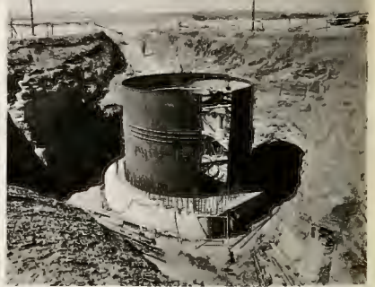
Steel wall rises above second elevation of missile launcher.
