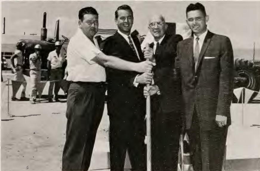
BUILDERS, main tenant and leasing agency all are represented in photo at right, clasping a groundbreaking shovel in a cooperative spirit. From left are Webb Project Supt. Frank Kelleher, Vice-Pres. Richard M. Wartes, Banker Cale Carson and Gene Hinkle of the Walker and Hinkle leasing firm. Said Mr. Carson at the ceremony: "This is a big day and a big project for Albuquerque." His bank leased the square block site to the Webb firm for 99 years and is leasing from Webb some 22,500 square feet of space in the new building. Jack Hummer of the Phoenix office is chief of project operations, Roland Beaulieu is project engineer and Jim Benson office manager.
