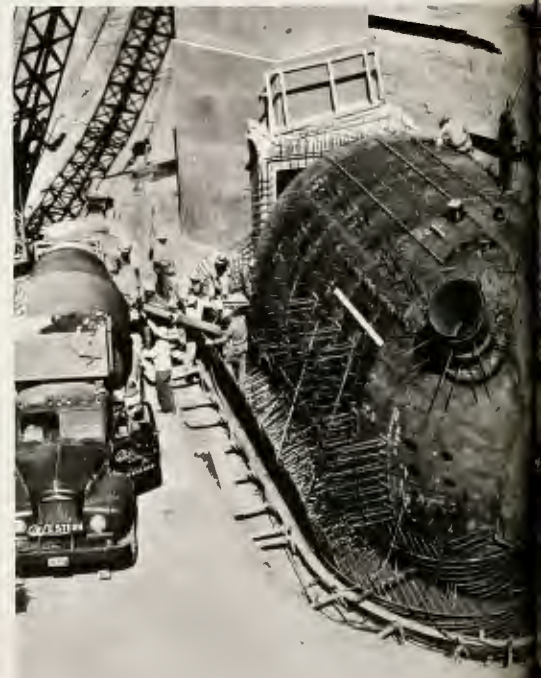
Launch control center begins to take and steel elevator shaft. Once concrete is ready for the egg-shaped, steel-enclosed capsule, it will be buried far below ground level when the U. S. Army Corps of Engineers).
