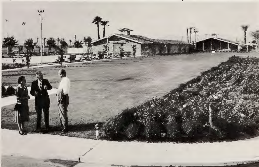
IN GARDEN-LIKE SETTING , this is the $250,000 recreational and community center presented by Webb Corporation to Sun City residents, who now assume responsibility for its operation and maintenance.
