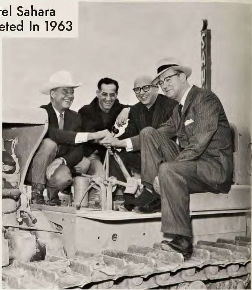
PLENTY OF TALENT was at the controls for the official ground-breaking to launch construction of the 24-story skyscraper addition to Hotel Sahara at Las Vegas, Nevada. Pictured above, from left: Rex Bell, Nevada's lieutenant governor; Alex J. Shoofey, Sahara-Nevada Corporation executive vice-president; Milton Prell, Sahara-Nevada president, and Del E. Webb, Webb Corporation president.
