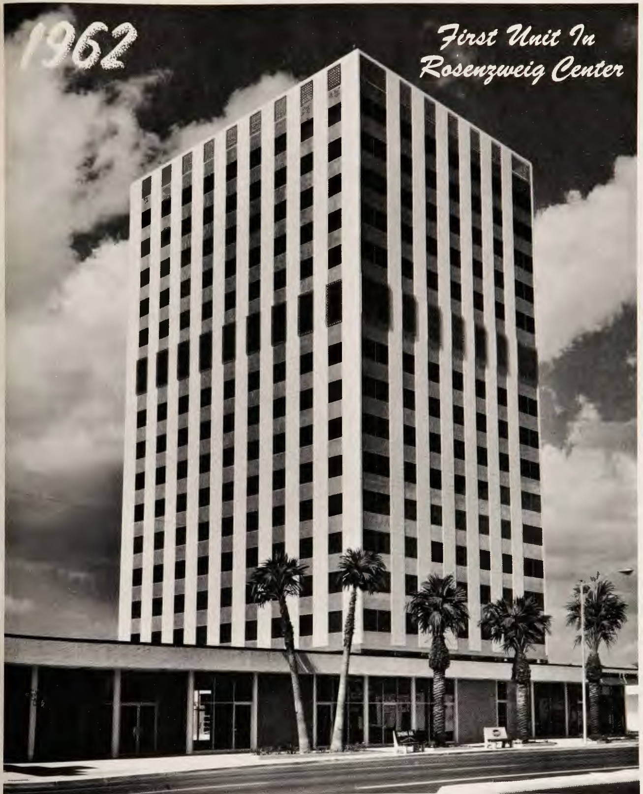
THE DEL WEBB BUILDING , sleek and modern, gold and white 17-story office structure on Phoenix' busy North Central Avenue, was completed and occupied in 1962. It became not only the corporation's home office, but also the first unit in the multi-million dollar Rosenzweig Center business complex to rise on 12½ acres the Webb firm controls at the prestige location. Besides scores of tenants in the building, ground floor space has been leased to a stock brokerage firm, title company, branch bank, jewelry store, travel agency, shoe store, haberdashery, beauty shop, office supply store, restaurant and cocktail lounge.
