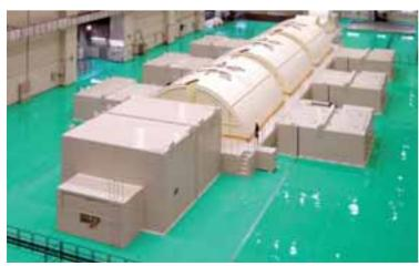
Hamaoka Power Plant Unit No.5 (Japan) 1380 MW, TC6F-52, 1800rpm 6.69 MPa, 284/253°C
