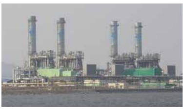
SK Power (Korea) 200.9 MW x 2, TCDF-40, 3600rpm 12.7 MPa, 565/565°C
