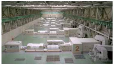
Kawagoe Thermal Power Station (Japan) 85 MW x 7, TCDF-26, 3600rpm 10 MPa, 538/538°C
