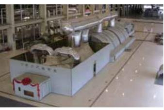
Zouxian Power Station Unit No.7 and No.8 (China) 1000 MW , TC4F-43, 3000rpm 24.9 MPa, 600/600°C
