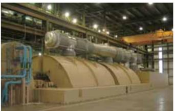
Water Scott, Jr. Energy Center No.4 Unit (USA) 870 MW , TC4F-40, 3600rpm 25.3 MPa, 566/593°C >>2007 Plant of the Year / Power-USA< >>Best Coal Fired Projects of the Year Awards 2007 / Power Gen International <<
