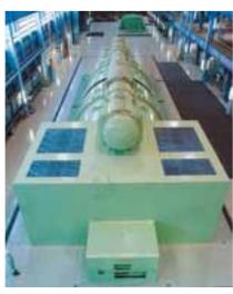
Tomato-Atsuma Power Station No.4 Unit (Japan) 700 MW, TC4F-43, 3000rpm 25.0 MPa, 600/600°C
