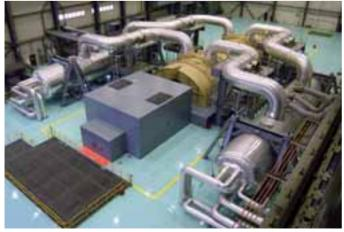
Qinshan III Power Plant Unit No.1 and No.2 (China) 728 MW, TC4F-52, 1500rpm 4.41 MPa, 257.6/243.4°C
