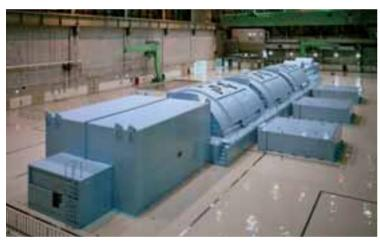
Kashiwasaki Kariha Power Plant Unit No.4 (Japan) 1100 MW, TC6F-41, 1500rpm 6.55 MPa, 282°C
