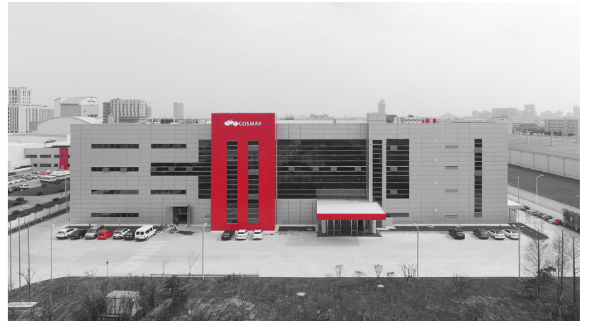
New Plant in Shanghai, 2017
