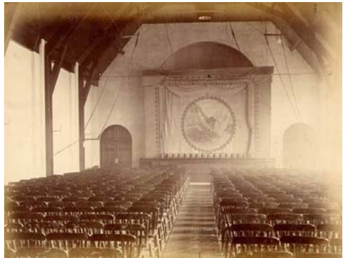
The main hall in 1890 & 2004, and new trusses in place in 2011.
