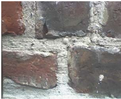
Lime pointing with beach sand, complete with shells!
