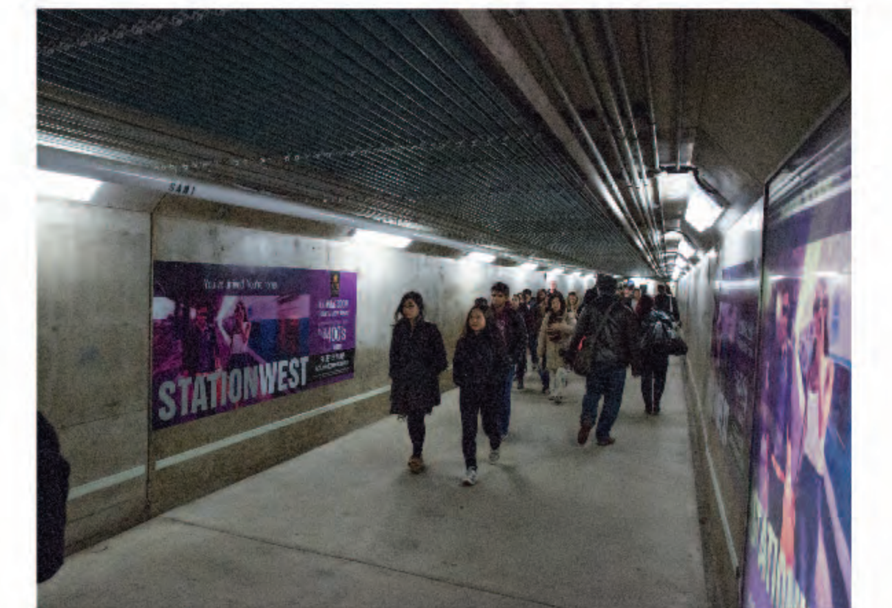
Example of underpass
