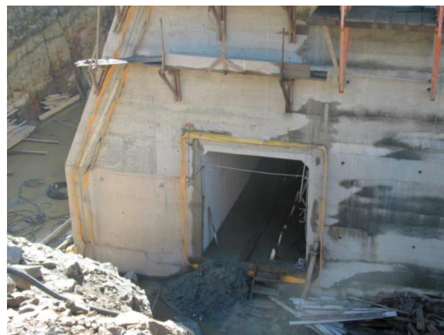
Photo 3 - Gallery of the RCC Dam
