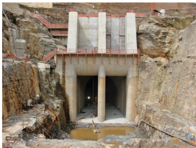
Photo 7 - Diversion Intake Structure before Diversion of the River
