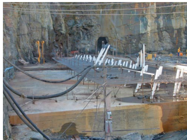
Photo 4 - Installation of Tubes for the Grout and Drainage Curtain
