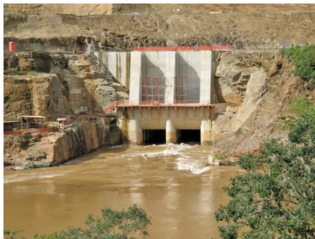
Photo 8 - Diversion Intake Structure in Operation
