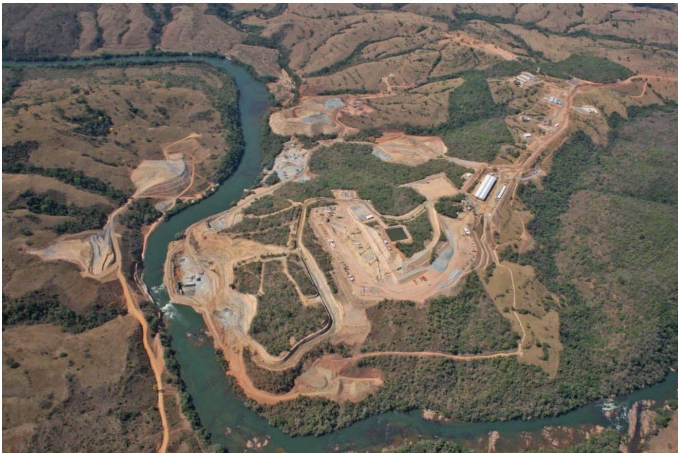
Photo 12 - Aerial View of the Diversion Works and Jobsite
