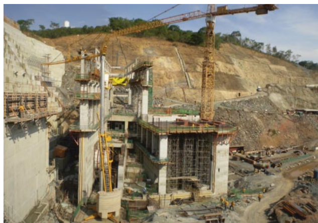
Photo 10 - Works in the Powerhouse - November 2008
