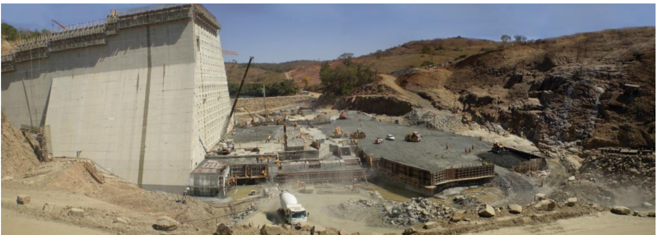
Photo 1 - Works on the RCC Main Dam seen from Upstream - August 2008
