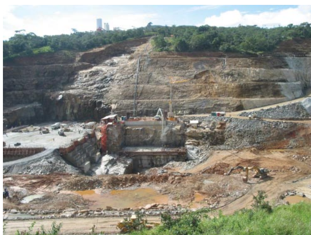
Photo 6 - Works on the Main Dam and Powerhouse - March 2008
