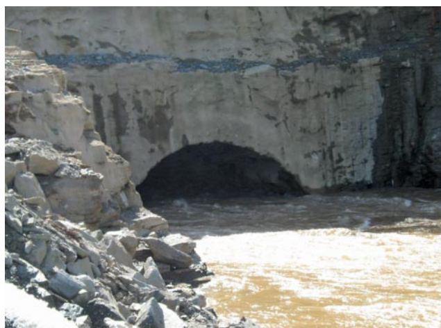
Photo 9 - Diversion Tunnel Outlet
