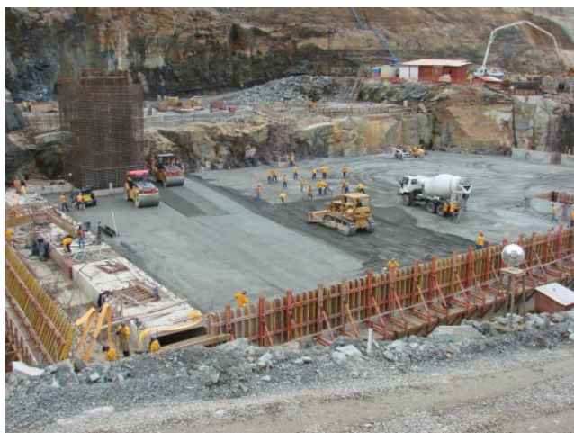
Photo 5 - First Layers of Rollcrete on the Main Dam - March 2008
