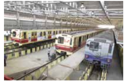
Carshed of Metro Railway at Kavi Subhash Station
