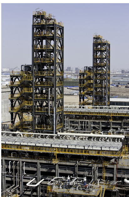
Ningxia Hanas Natural Gas Co. Ltd., Ningxia, China plant utilizes Air Products' single mixed refrigerant (AP-SMR™) process.
