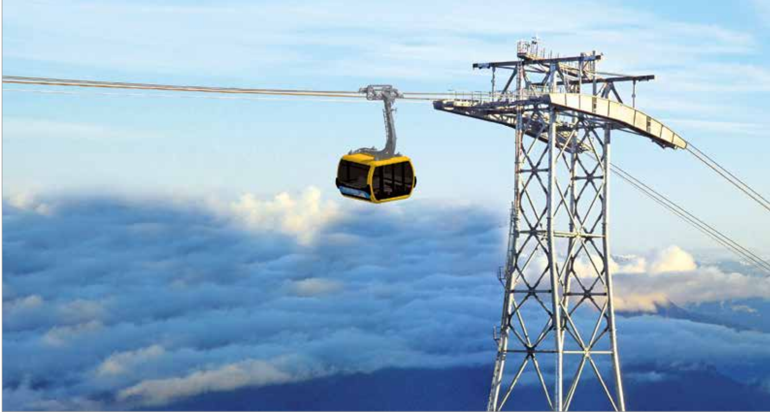
Anyone who is interested can follow the progress of the construction of the new Penkenbahn in the online report at www.mayrhofner-bergbahnen.com .
