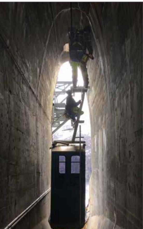
Work on the aerial tramway in the tunnel.
