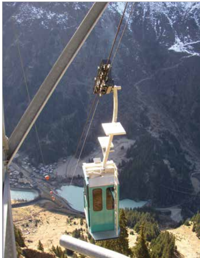
An aerial tramway grants access to the surge chamber for fast, weather-independent troubleshooting at the installations of the storage power plant.
