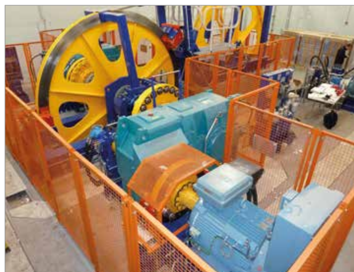
Below the surface, the fanciful fairytale train is technically speaking a cable liner with its time-tested, reliable drive system.
