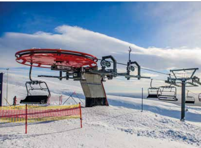
In the winter of 2013, BMF built its first line in Kirovsk, a fix-grip quad chairlift spanning 1.066 meters (3,500 ft.). Left: The two stations.
