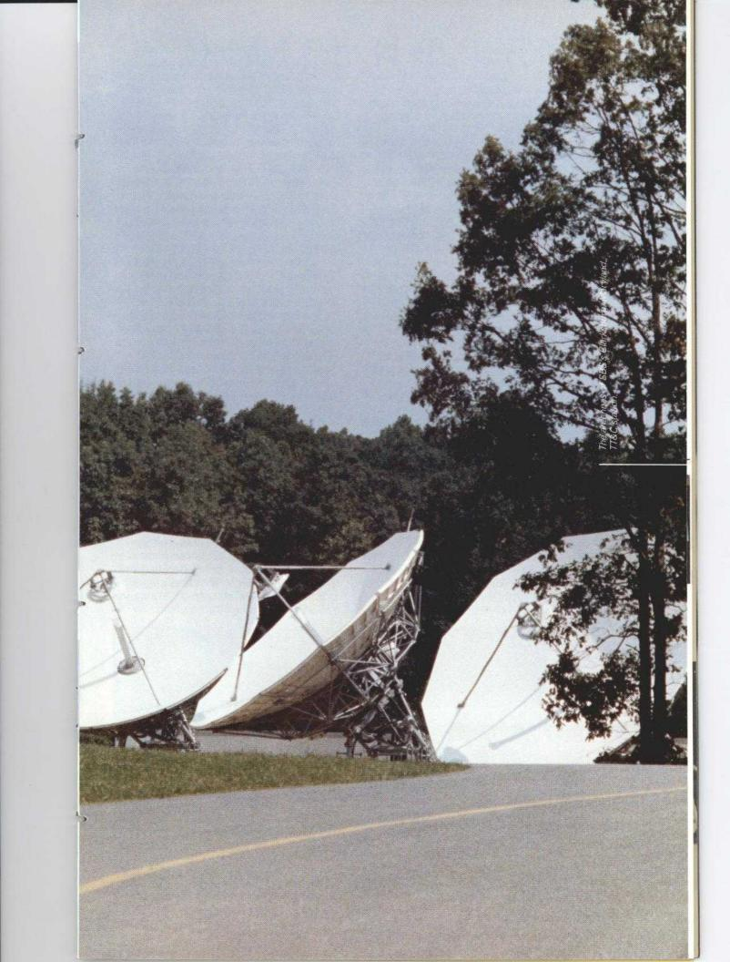
of a car—without which, the seemingly more important parts (the motor or transmission) lose their value. Working in concert, forming a triangle with the satellite, the stations will track and steer the satellite, keeping it within a small "box" in space.
