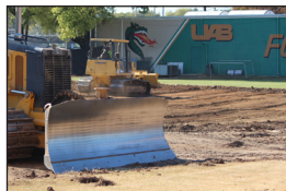
Construction on the first of two turf practice fields begins. Once completely finished, the entire facility will have two turf fields and one grass field.
