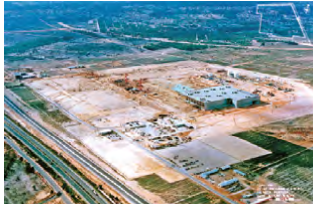
PALMELA PLANT SHELL CONSTRUCTION
