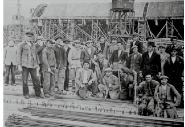
ITALIAN CONSTRUCTION WORKERS AT THE MAIN PLANT
