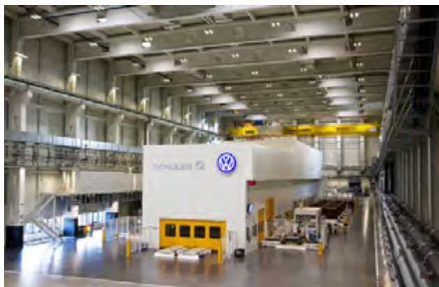
PRESS PLANT IN BRATISLAVA
