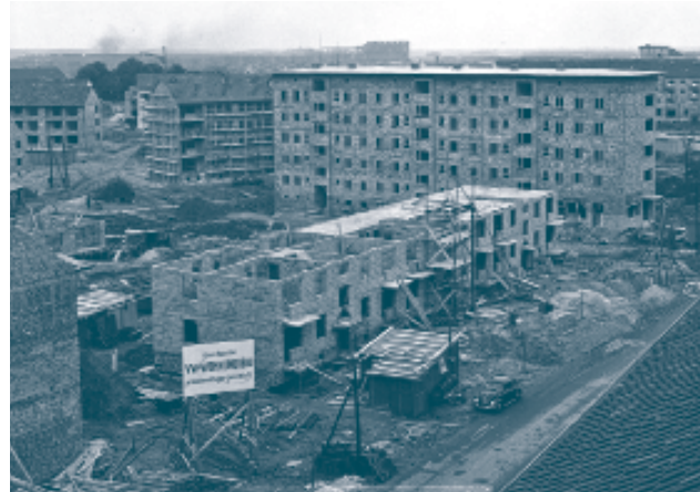
CONSTRUCTION OF COMPANY HOUSING IN WOLFSBURG
