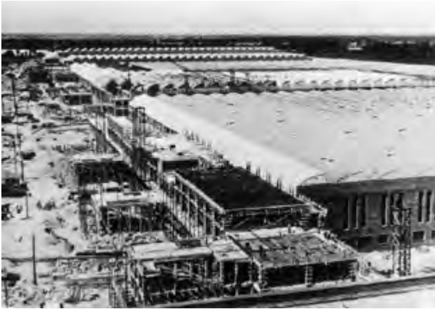
MAIN PLANT SHELL
