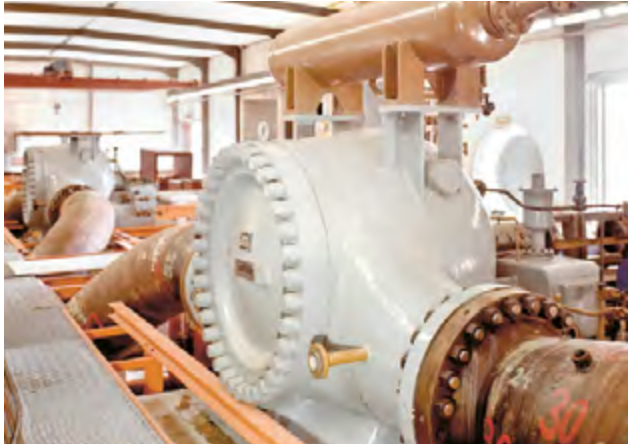
TURBOCOMPRESSOR
