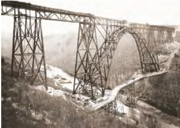
CONSTRUCTION OF THE MÜNGSTEN STEEL BRIDGE
