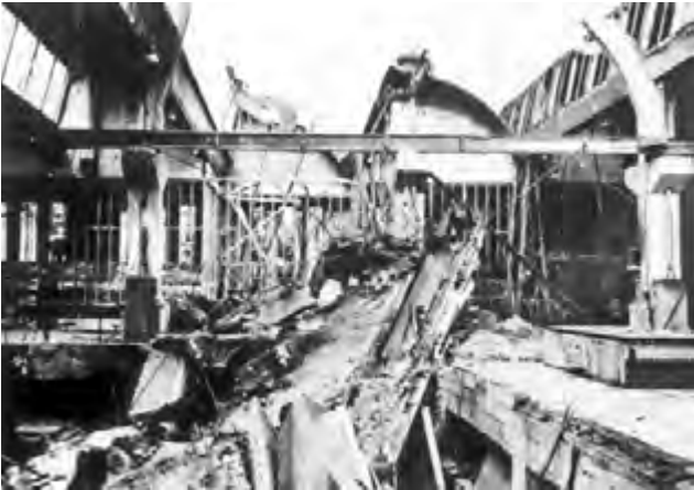
BOMB DAMAGE AT THE MAIN PLANT
