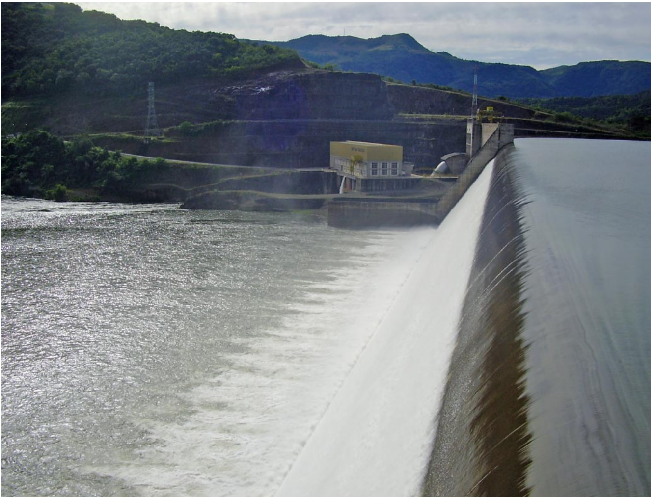
Photo 2 - Dona Francisca Spillway in Operation
