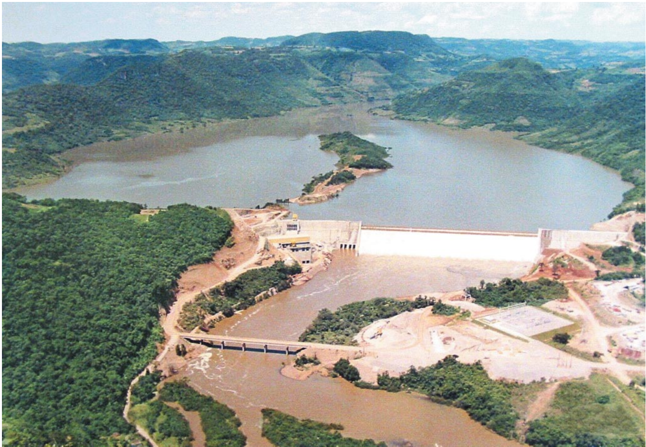
Photo 1 - Dona Francisca HPP - General View
