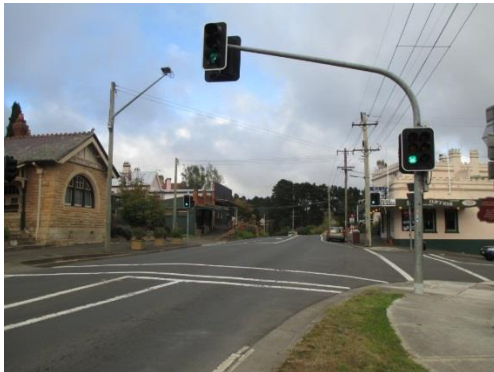
Great Western Highway/Station Street
