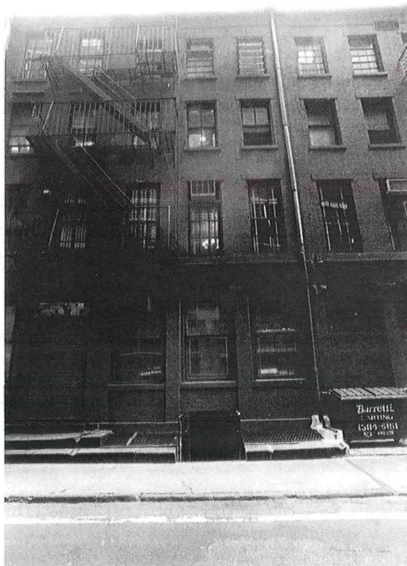
Nos. 99-101 Pearl Street, Hanover Bank Building Photo: David Breiner
