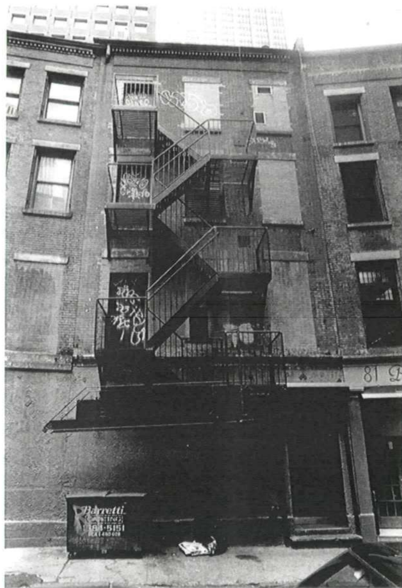
No. 50 Stone Street, aka 83 Pearl Street Photo: David Breiner
