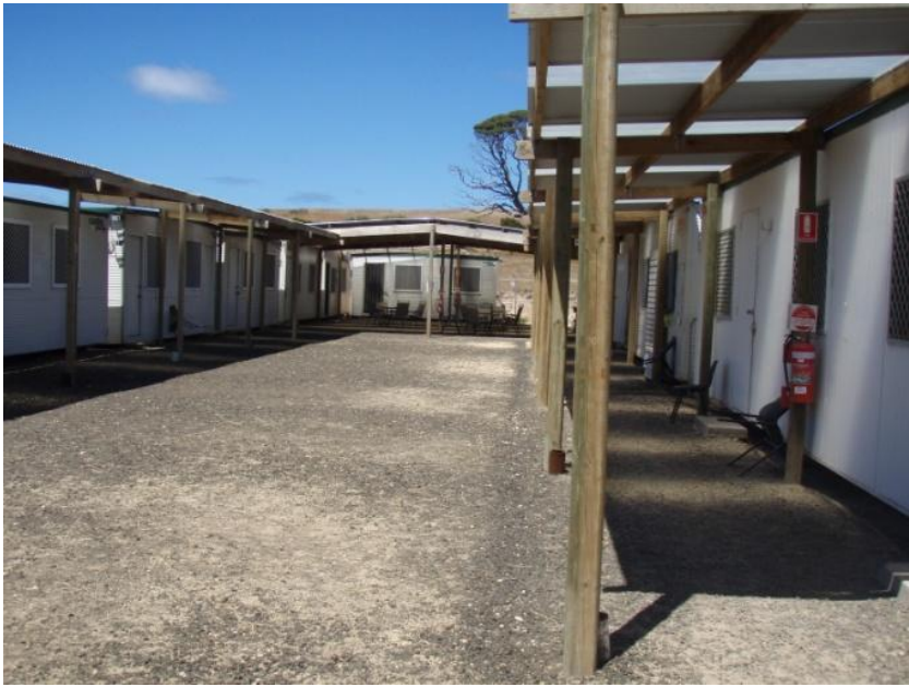
Photo 3.5: Site Offices within Temporary Compound (from Cape Bridgewater Wind Farm)
