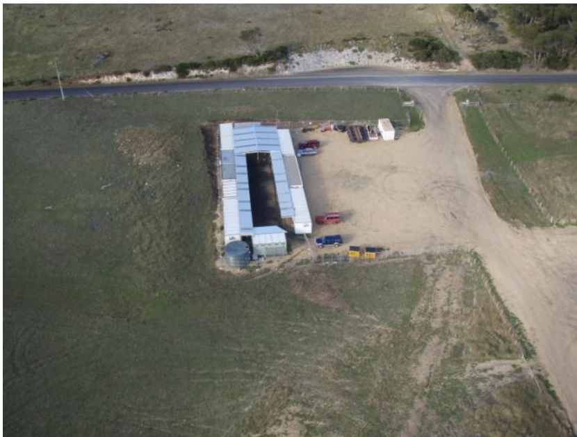
Photo 3.4: Example Temporary Compound (from Cape Bridgewater Wind Farm)
