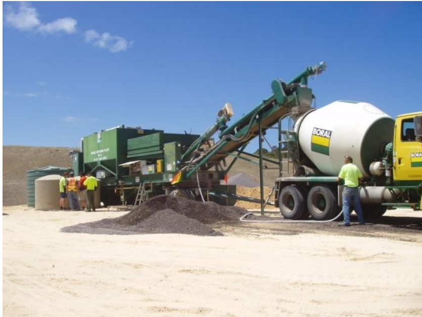
Photo 3.6: Example Batching Plant
