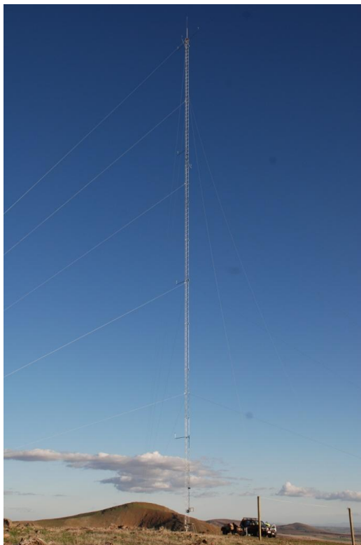
Photo 3.3: Indicative Meteorological Mast Appearance
