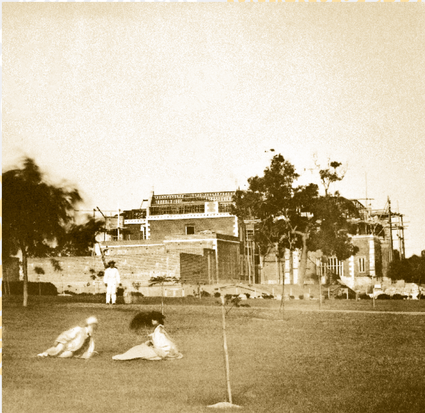
ABOVE: Government House under construction 1862. State Library of Western Australia 6293B.14
