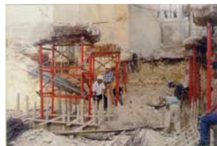
Figure. 1 Previous Underpinning Procedure in Ashrafieh, Lebanon
