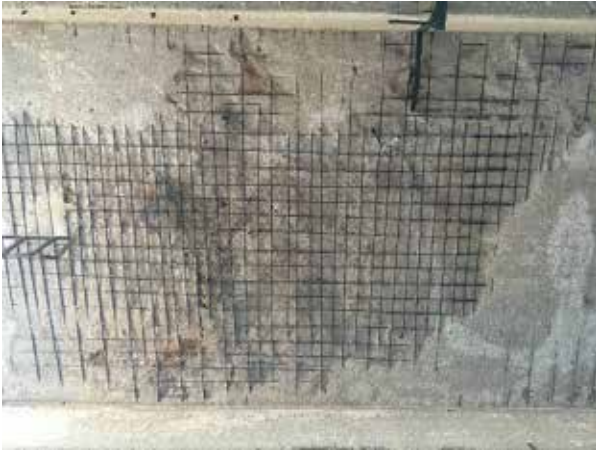
Figure 3: Spalled slab.
