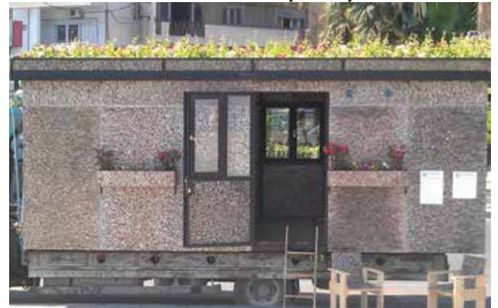
The prefabricated house
