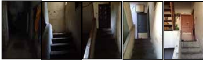
Figure 5. Pictures showing the change in the level of daylight in the building
