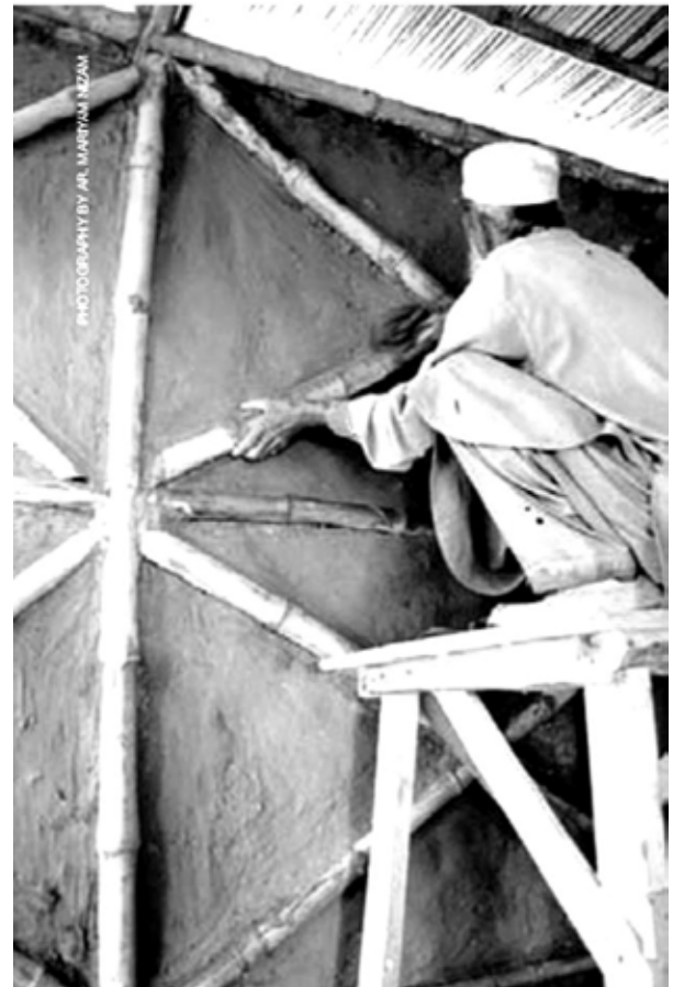
Fig. 6. Split bamboo planking used for roofing [7]
