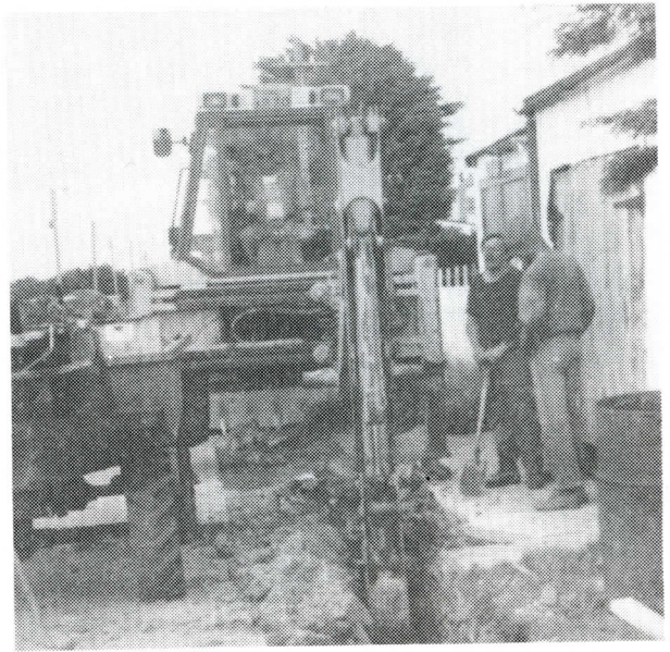
DIGGING THE DUCTS IN STANLEY (photo: R. N. Spafford)
