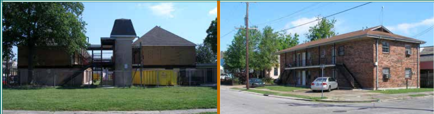
Existing Scattered Site - Mazant Royal Property
