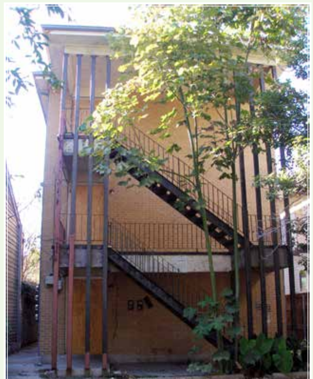
Existing Scattered Site - 1421 Constance Street
