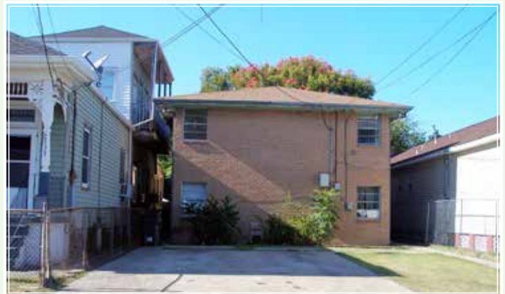
Existing Scattered Site - 2331 Annunciation Street
