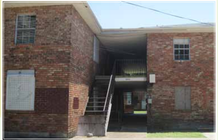
Existing Scattered Site - 2522 N. Rampart Street
