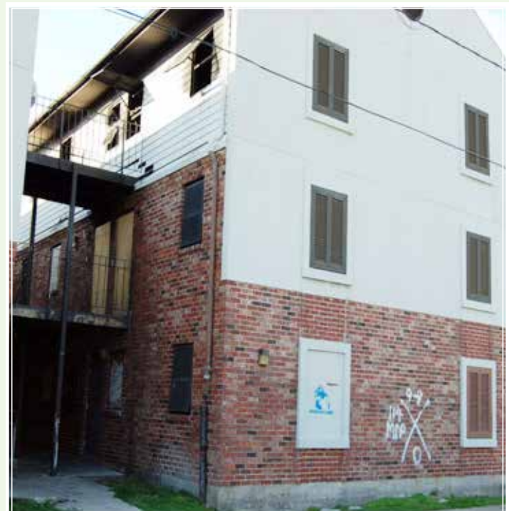
Existing Scattered Site - 1229 Constance Street
