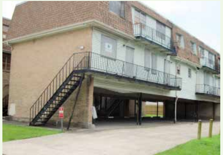
Existing Scattered Site - 5312 Constance Street
