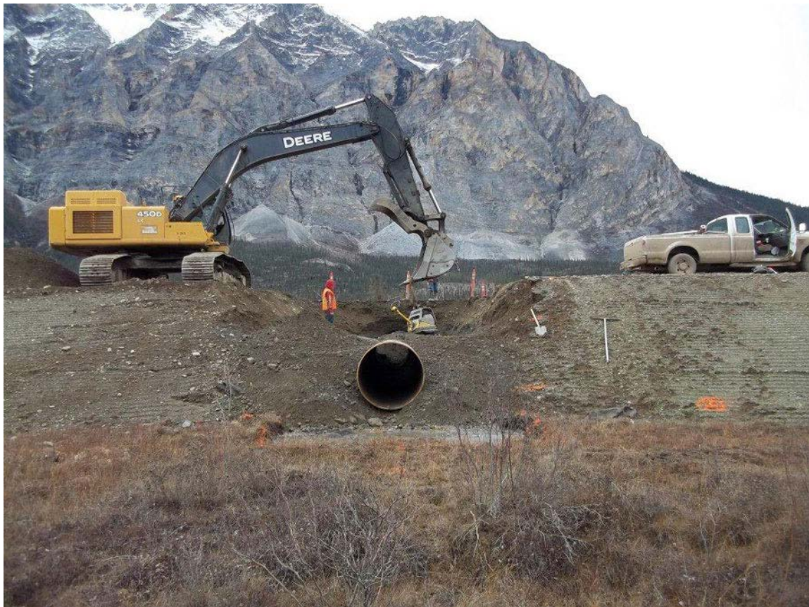
Culvert work, Dalton Highway Photo by Travis Donovan, Alaska DOT&PF
