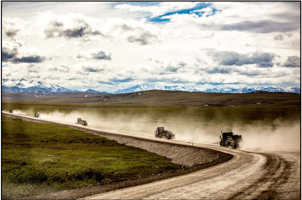
Dalton Highway MP 274-289, near the Kuparuk River
