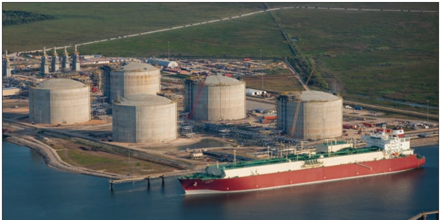
The Golden Pass liquefied natural gas terminal in Sabine Pass, Texas, initiated commissioning and achieved first gas send-out in 2010. The diversity of our gas portfolio and global presence allows us to maximize value through access to many markets.
