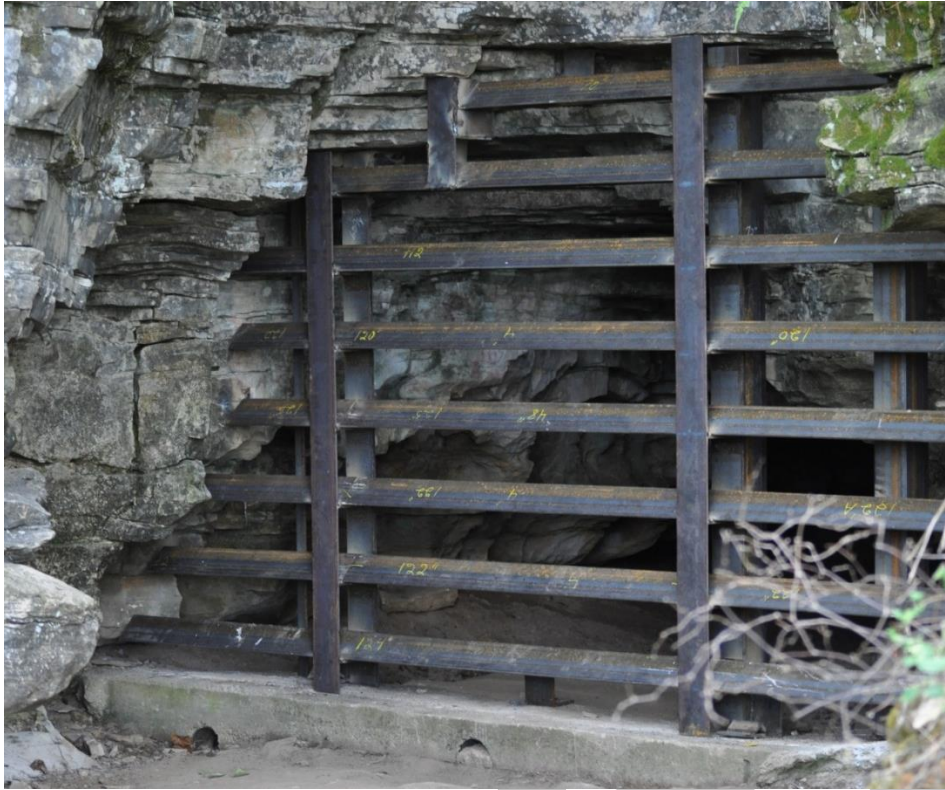
Figure 9 The new gate, installed in 2012, reflects current bat-friendly gate standards.
