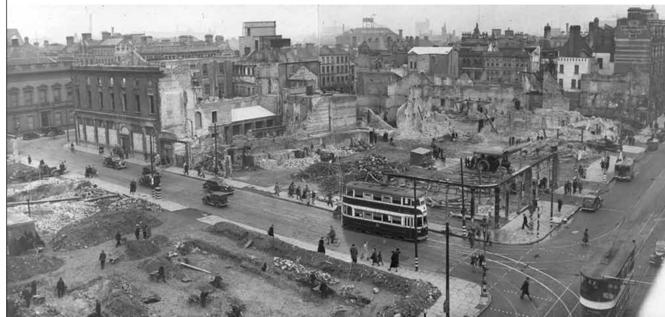
'Blitz Square' (the corner of Bridge Street and High Street) following the air raid of May 1941. The photograph shows that few of the nineteenth-century buildings in the centre of Belfast have basements or cellars. This suggests that, if they were present, archaeological horizons of medieval date would survive relatively intact. The failure during the course of several excavations to find any significant evidence of medieval activity within this area, set between the known sites of the castle and the Capella de Vado (Chapel of the Ford), suggests that the main focus of medieval settlement was situated elsewhere within the immediate vicinity of the modern city centre.
