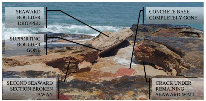
31 January 2014. Anastasia's Pool, viewed toward the sea. The concrete base, which was visibly damaged in the picture on the 21st January 2014 is now is no longer evident at all. The supporting boulder has disappeared, with the result that the seaward boulder has now dropped. A second seaward section of rock has also broken away. The remaining seaward side of Anastasia's Pool has a large crack at the wall/floor interface.
