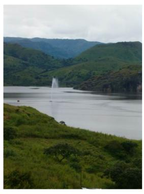
degassing The current project constitutes of a big pipe placed vertically into the lake. The water in the pipe has been initiated to flow vertically and has been kept flowing up since. As the water pressure drops, while the water flows up, the gas evaporates in the pipe causing the density to drop dramatically. Thus, the water is pushed upward by hydrostatic pressure and leaves the pipe at the top with high speed, causing a fountain up to some 50 meters high.
