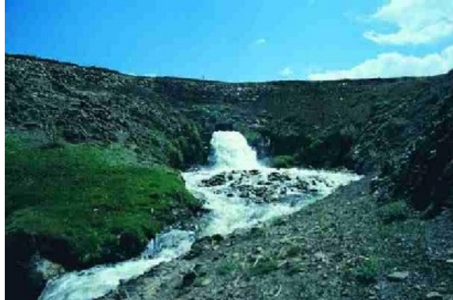
Fig. 6: A view the bottom sluice of Rusa Dam
