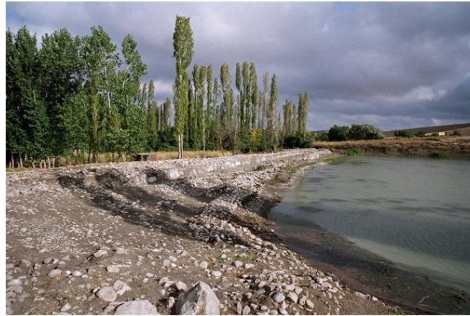
Fig. 1: A view of the Hittite dam
