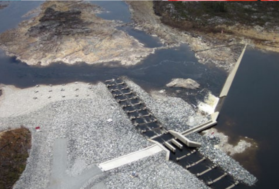
Fish pass built at KP 207 of the Eastmain (looking downstream)
