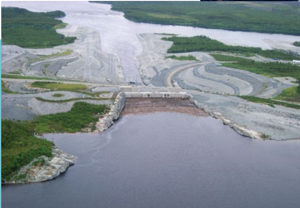
Wood debris at the Eastmain-1 powerhouse intake
