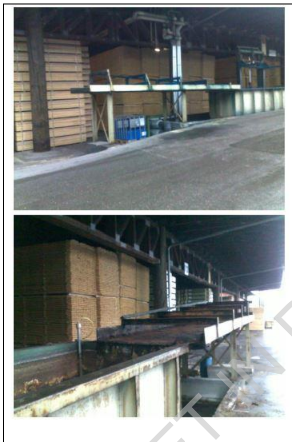
Figure 15.27: Example of a drip pad with dripping treatment solution flowing back into the treatment vessel
