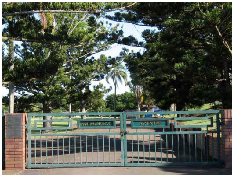
The entrance to the Memorial Avenue at Wynnum State High School (March 2006)
