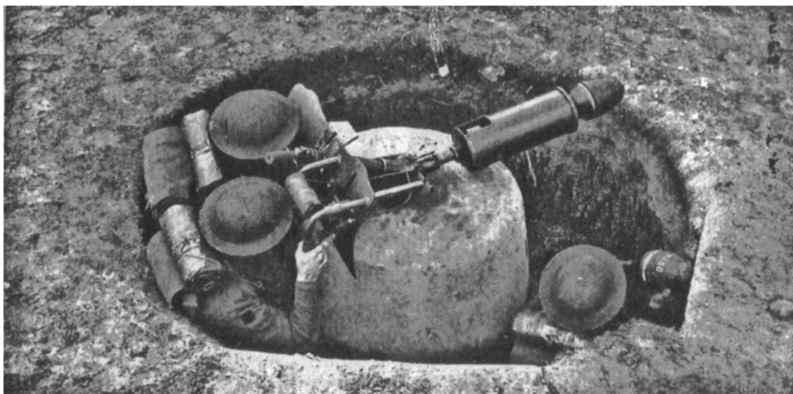
A Spigot Mortar detachment in position using a concrete pedestal mounting. The ammunition number (right) is removing a drill round from the concrete roofed ammunition store, another of which is situated to the bottom centre of the picture. From the manual of 1942. (Author's collection)
