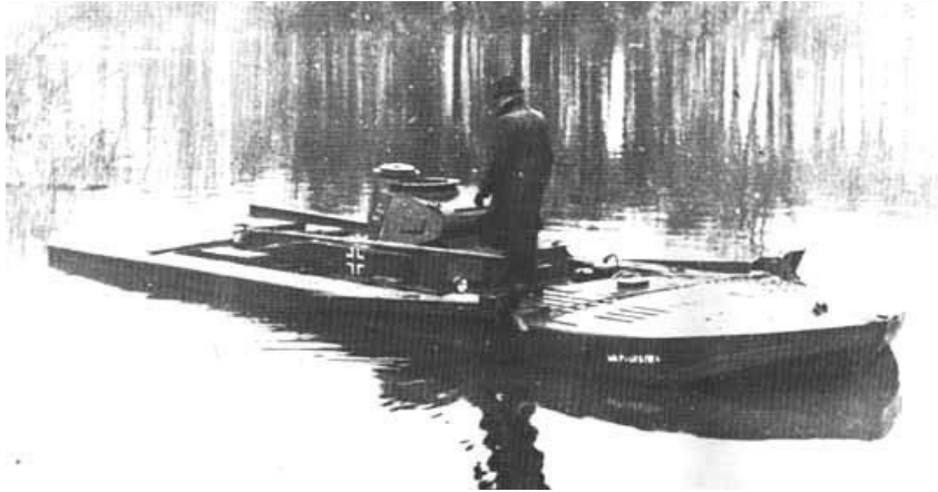
(Above): PzKpfw II amphibious variant fitted with boat-like buoyancy tanks, (www.odkrywca-online.pl)
