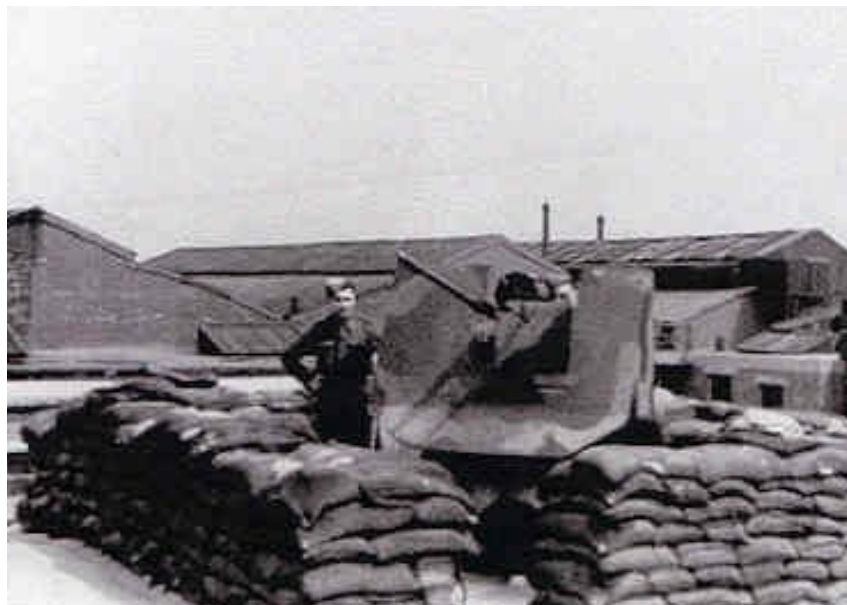
(Right) 20mm Hispano-Suiza (possibly the same gun) fitted with an armoured shield and emplaced on the roof of the factory fire station. (K. Musgrave, www.levyboy.com )
