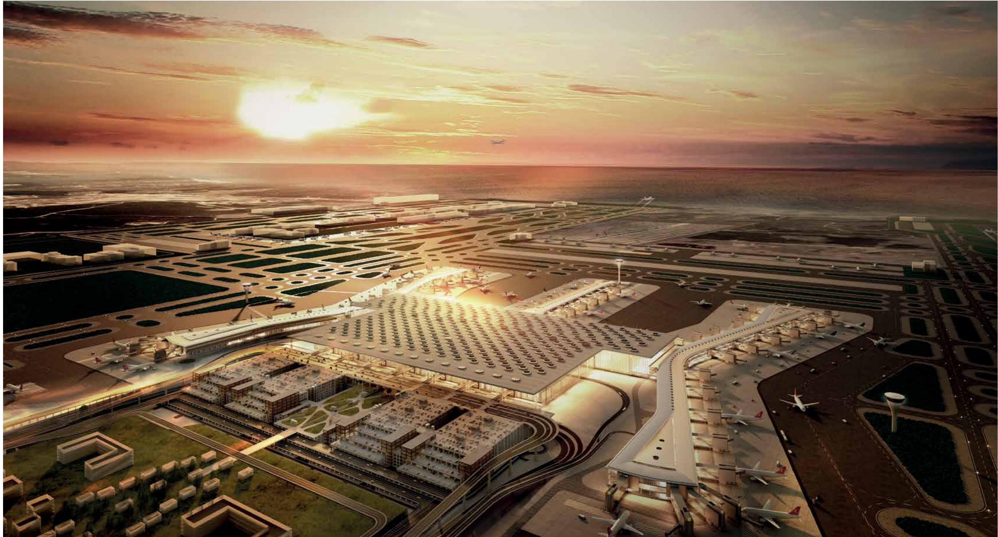
Istanbul New Airport Project, Phase I, Turkey
