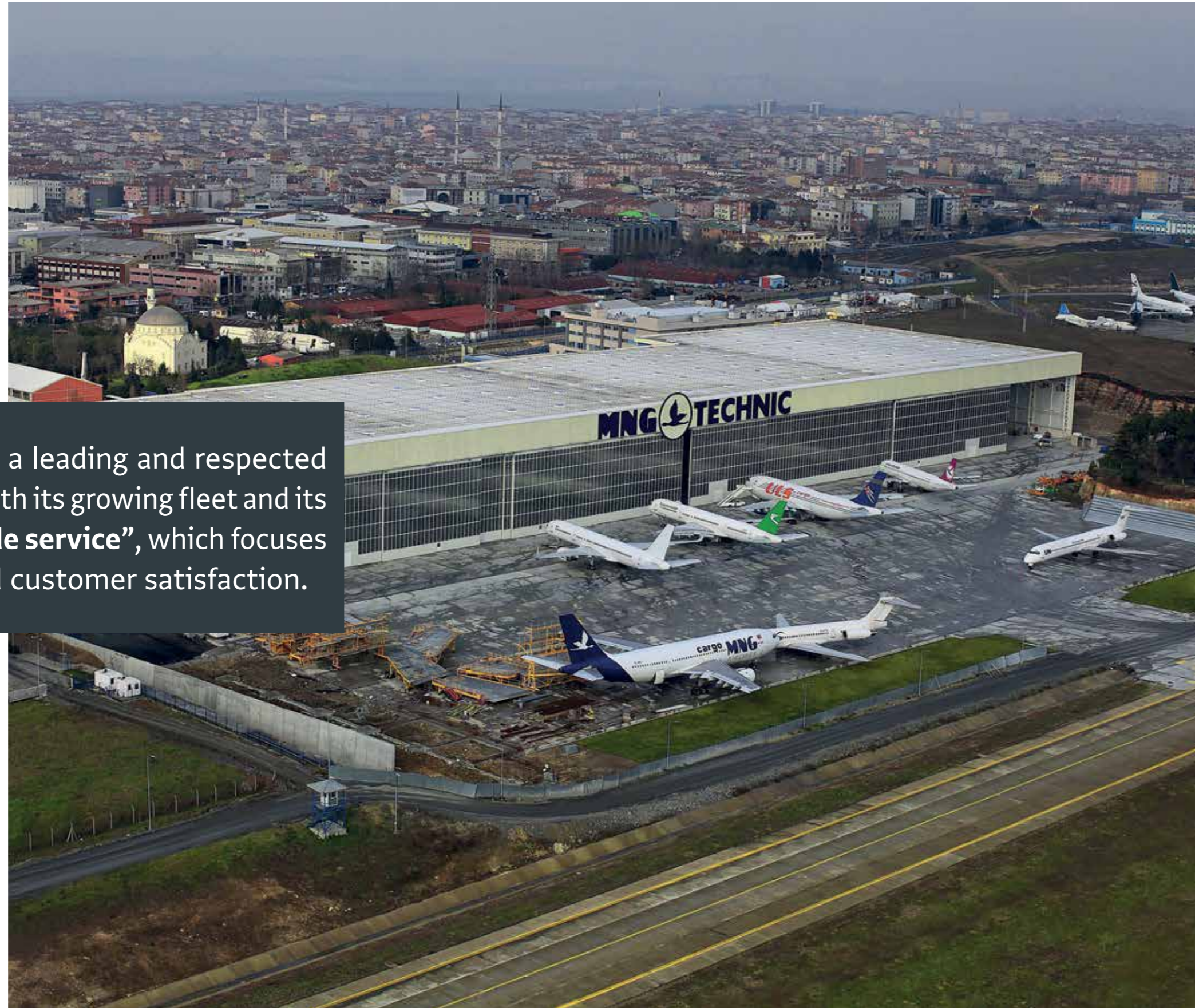
Aircraft Maintenance Hangar, Turkey
